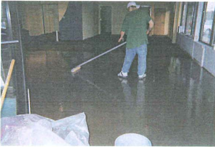
1. Applying ECO-POXI with 18" roller brush.
