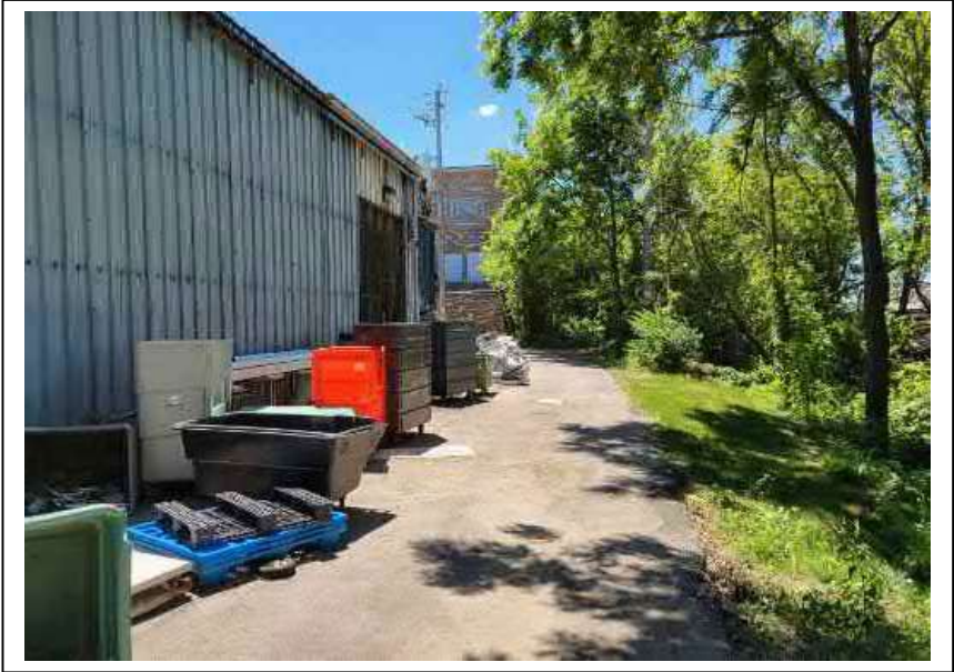
PHOTOGRAPH # 2 Taken on: 6/27/21 Description: View of engineered barrier along west side of building, facing south. Union Pacific Right-of-Way visible on the right side of the photograph.
