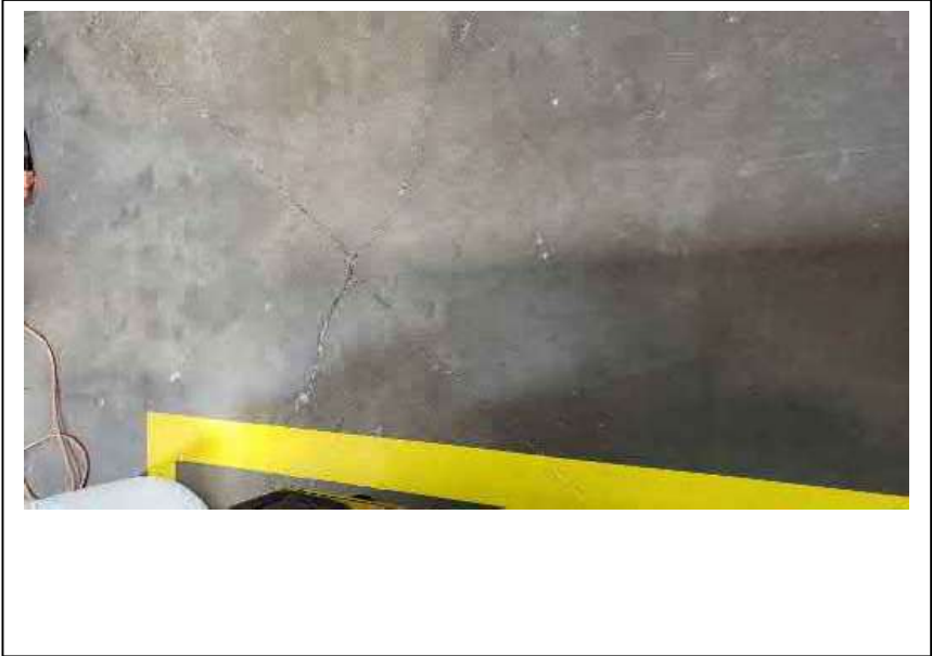
PHOTOGRAPH # 2 Taken on: 12/27/2021 Description: View of the concrete floor within southwest corner of the building.
