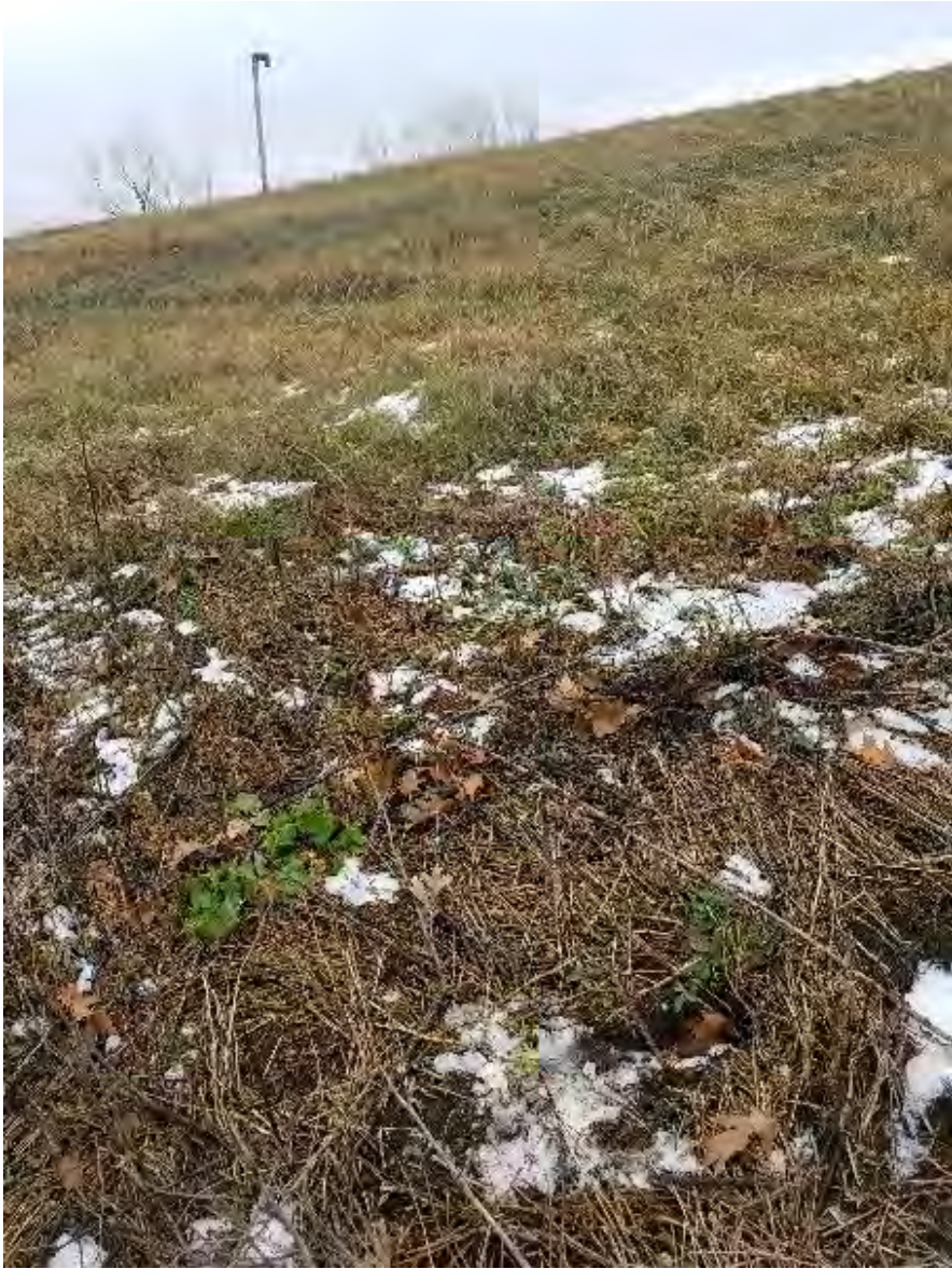
25. Bare spot in vegetation, looking uphill SE towards GV-2
