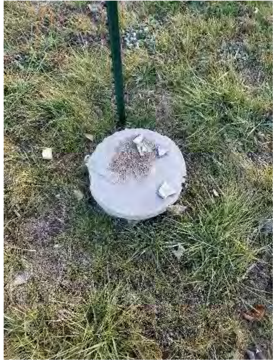
136. Broken cover of southern unmarked possible LHW by leachate piping
