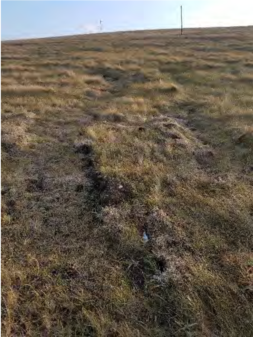
91. Slight erosion or tire tacks, looking S uphill towards GV-11
