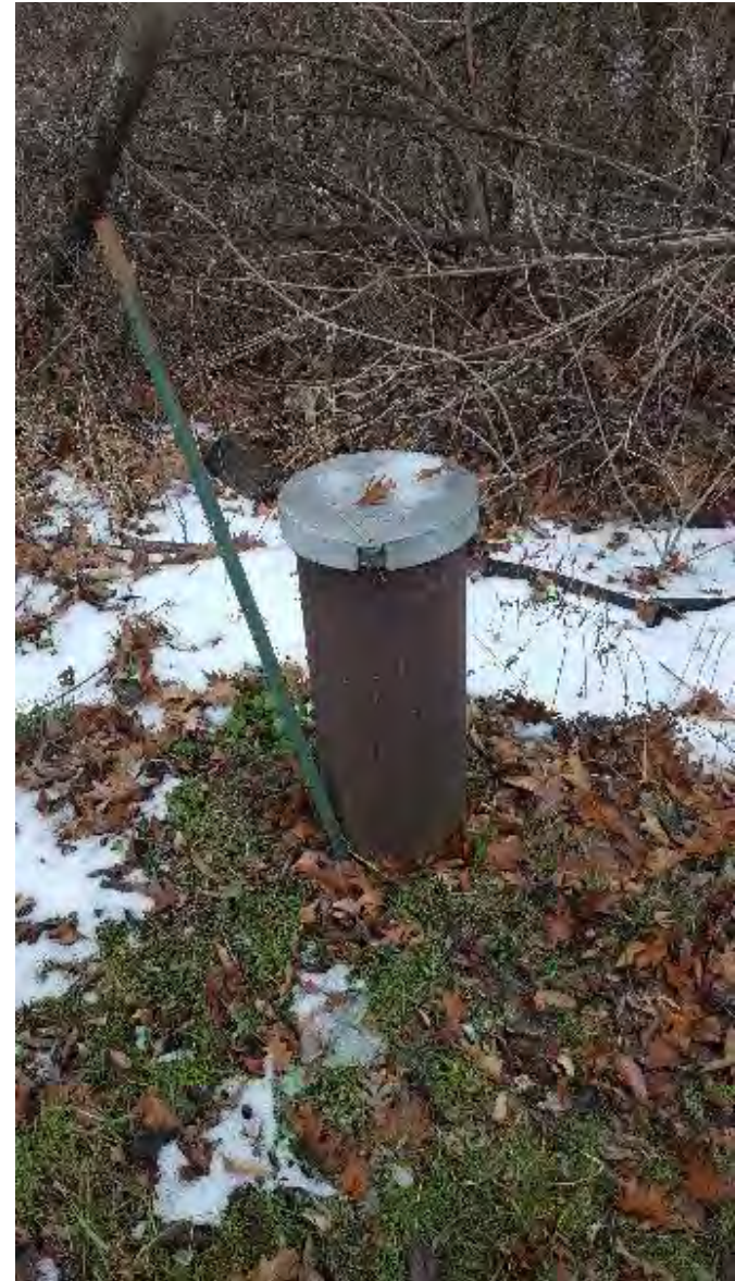
42. B-94-26 looking S, no lock
