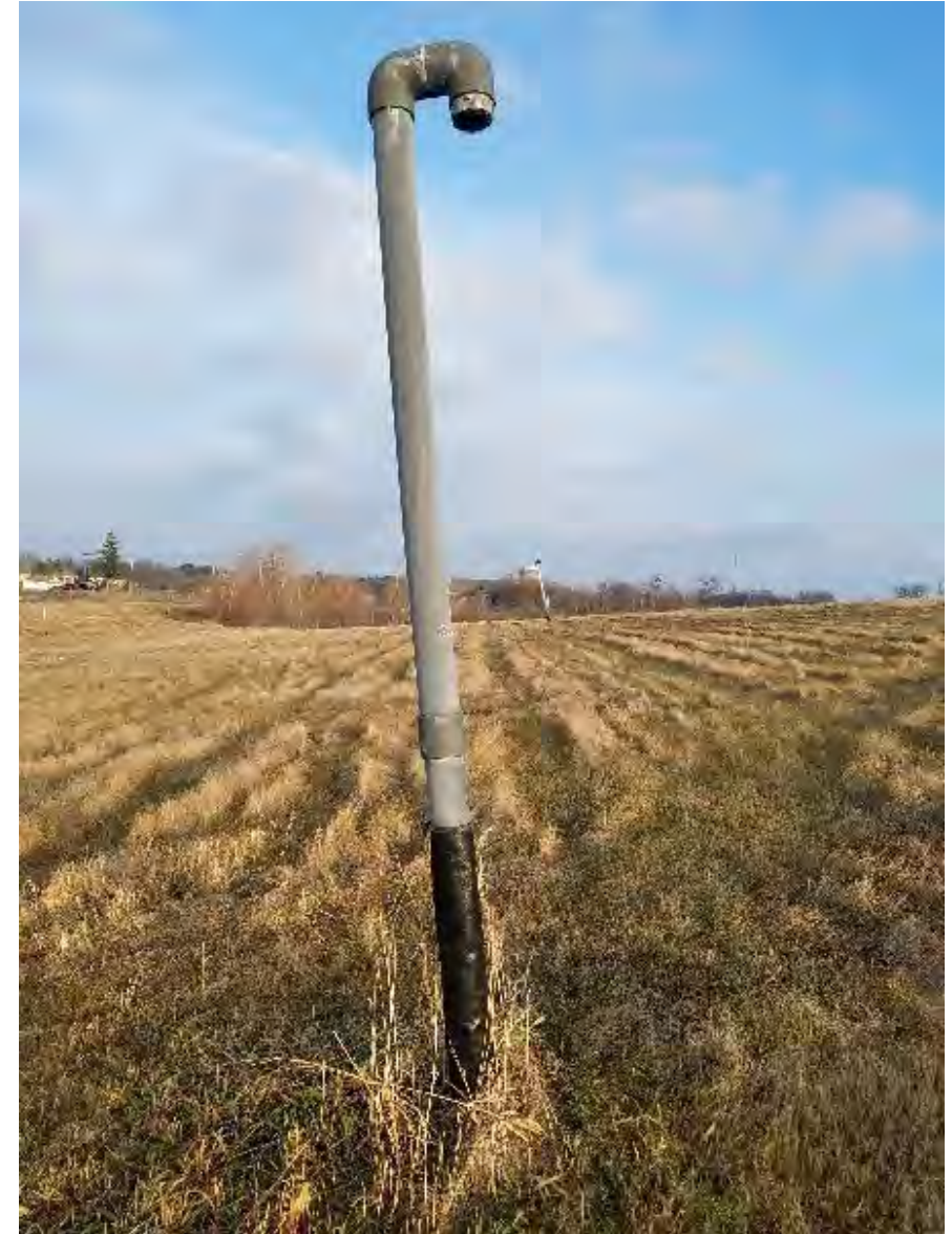
92. GV-12 slightly tilting N, looking E
