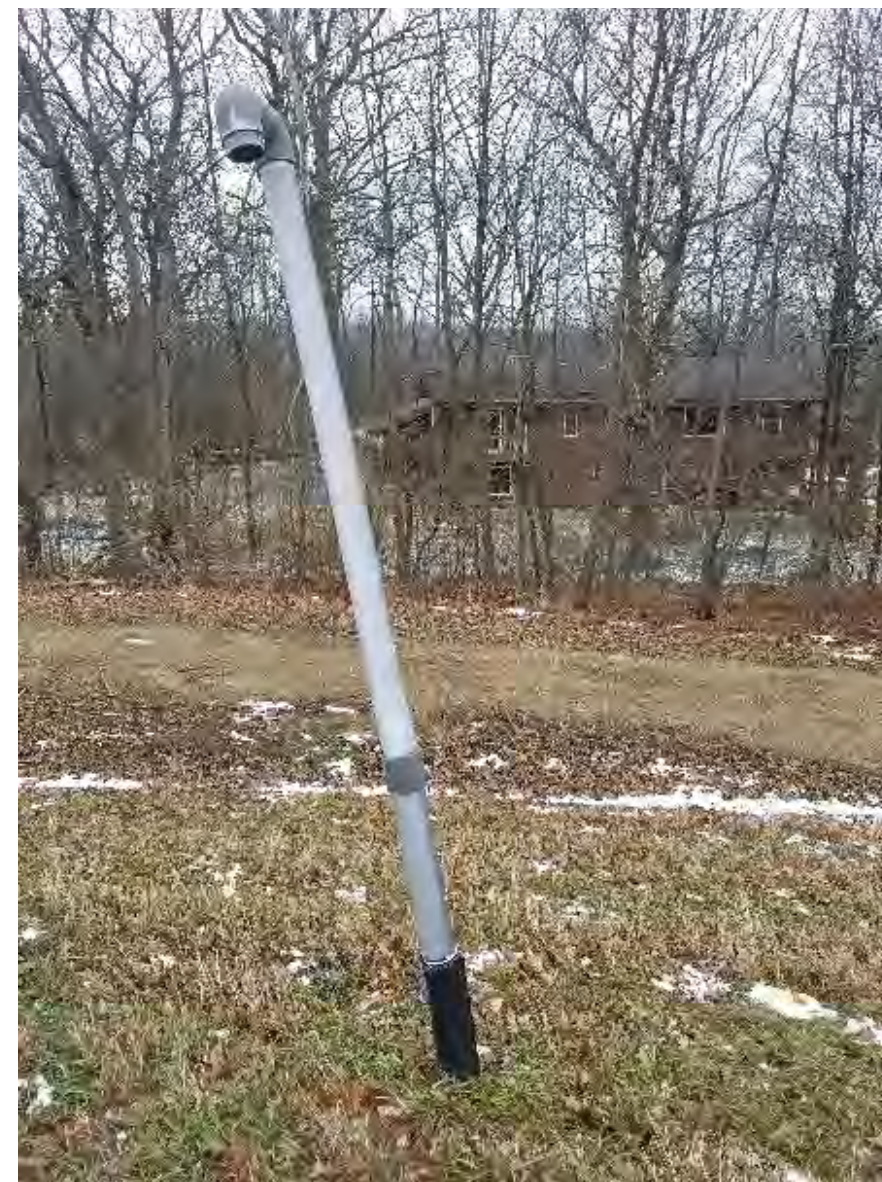
44. GV-47 tilting E, looking S towards Sanchez residence
