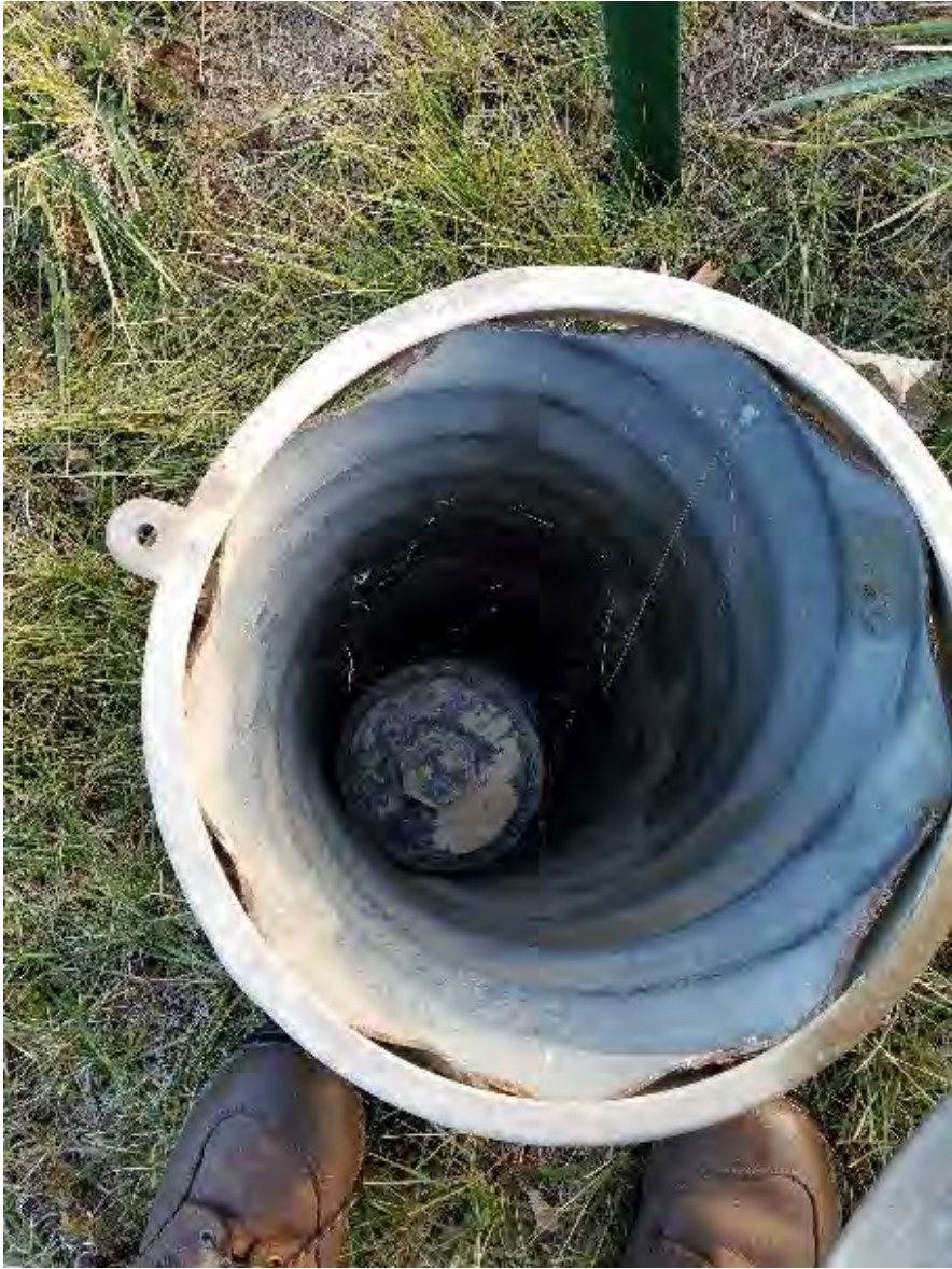
137. Inside unmarked southern LHW by leachate piping
