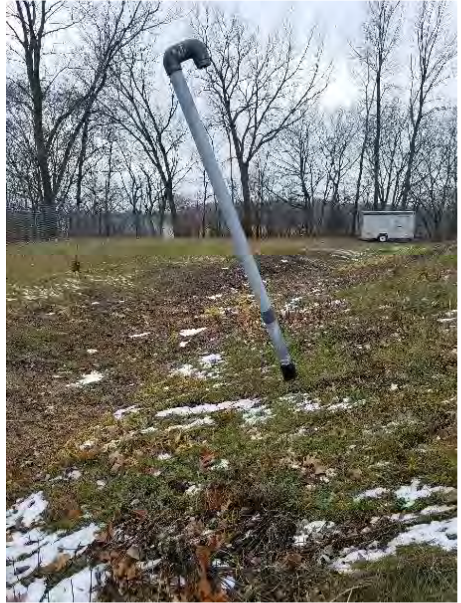
30. Unmarked GV tilting E, looking S at GP-9, towards SE corner of LF
