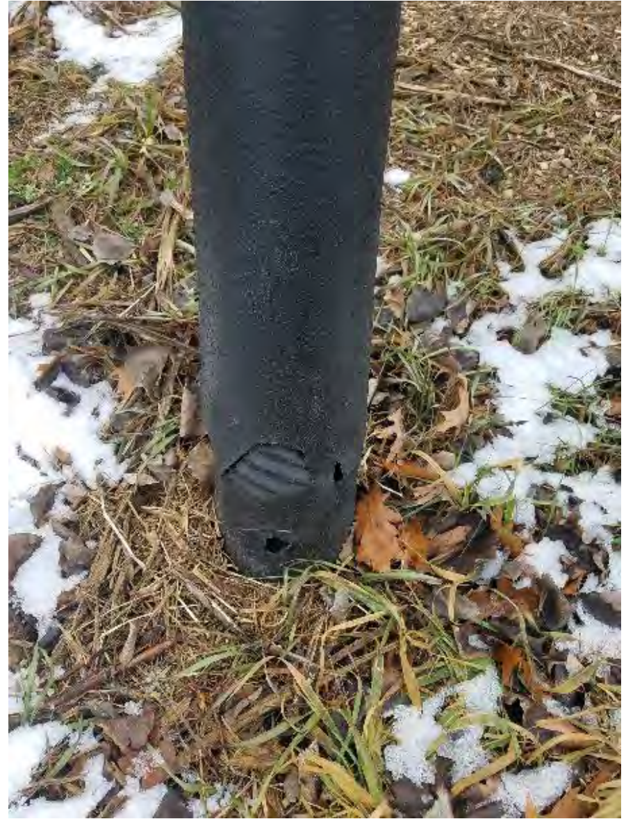
52. Tear in boot of un-numbered capped off LHW by GV-46
