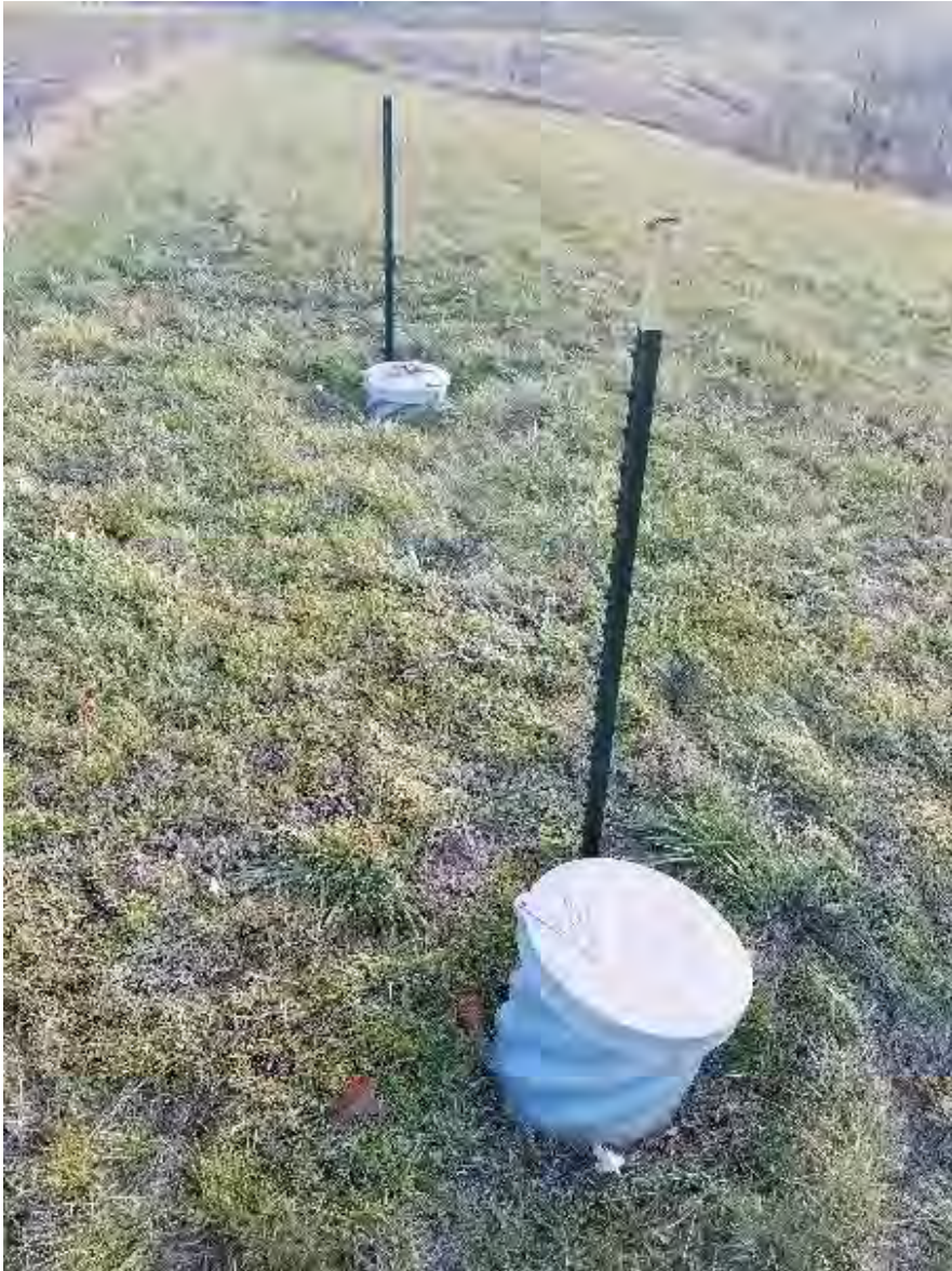
139. Possible LHW by leachate piping both unmarked, looking N
