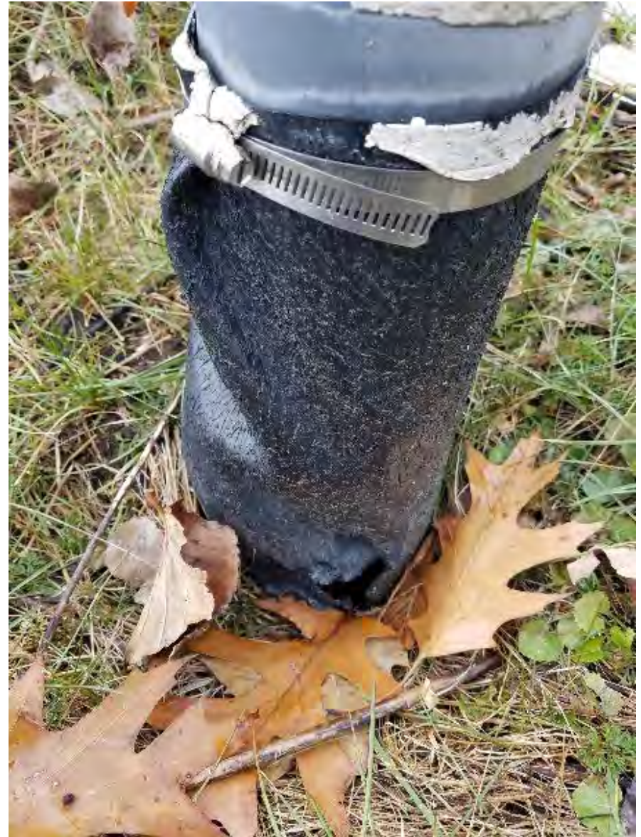
32. Unmarked GV by GP-9 damaged liner spot #2
