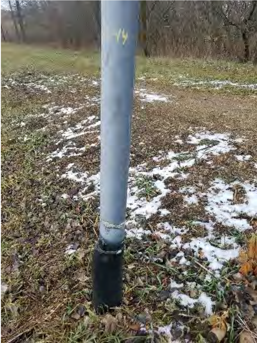
55. GV-44 looking SE at tightened hose clamp
