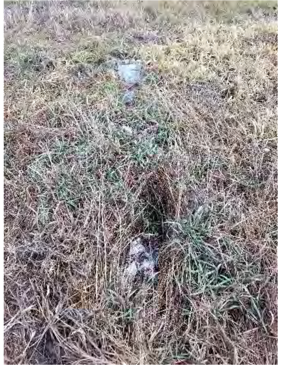
16. Damaged drain pipe
