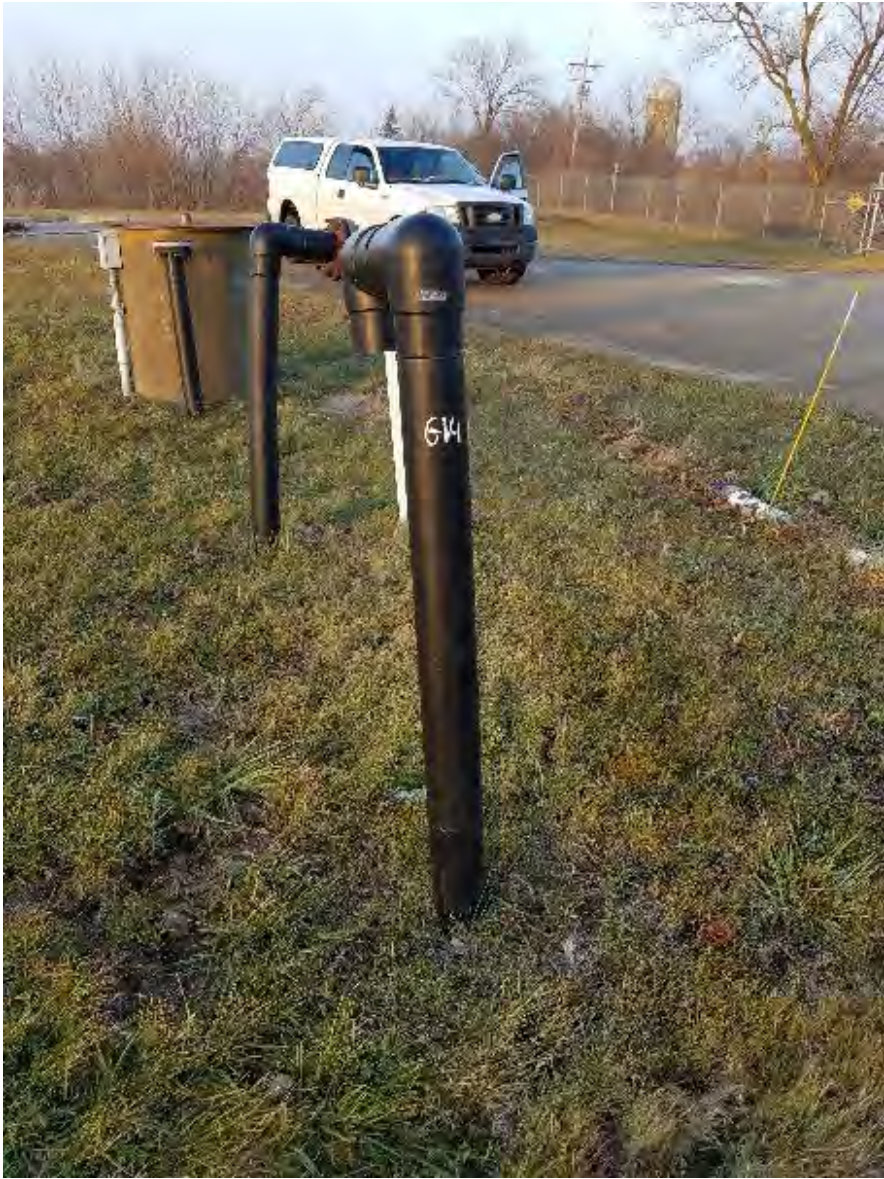
135. GV-1, looking S
