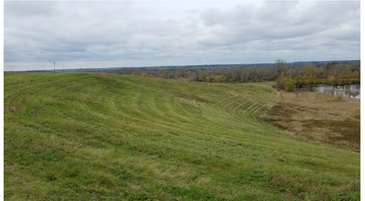
82. Site overview looking Northwest
