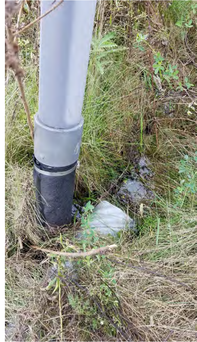
52. Drainage pipe at base of GV-123
