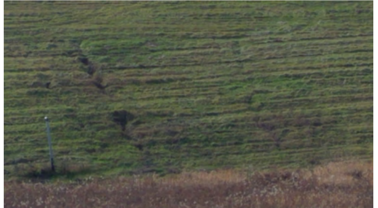
92. Extent of erosion down hillface #2
