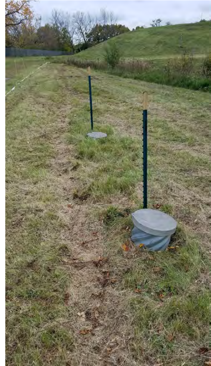
86. Unmarked vaults – possible parts of old leachate system
