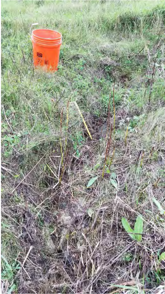
45. Erosion down hill face #2
