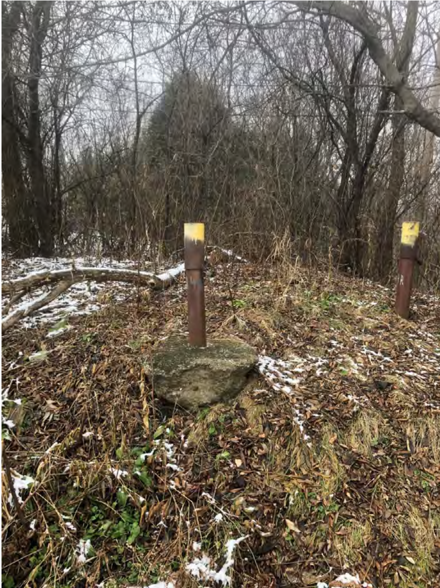
126. B-94-14A – eroding ground slope at base of well
