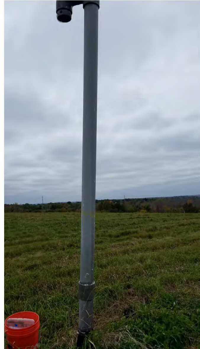
56. GV-122 Slight Northeast tilt
