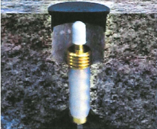
1. Vapor Pin installed through floor slab
