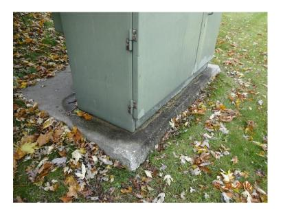
16. Minor staining on concrete pad for transformer on north side of former Denny's Restaurant building.
