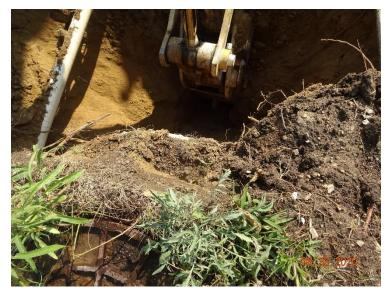
9. Excavating east of MH 2 with one (1) underground fiber optic utility exposed in the northwest corner of the Site.
