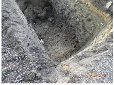
6. Compacted clay within the sanitary sewer trench west of MH 4 at the northeast corner of the Site.
