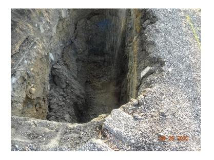
4. Backfilling sanitary sewer trench with compacted clay west of MH 4 at the northeast corner of the Site.
