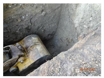
3. Excavating sanitary sewer trench west of MH 4 at the northeast corner of the Site.
