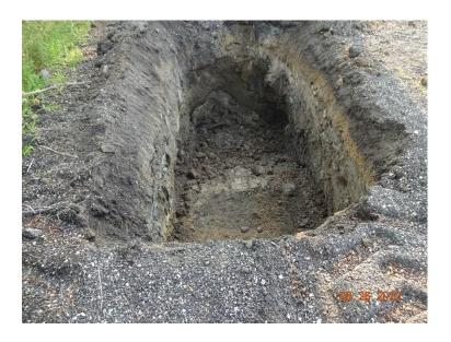
7. Compacted clay within the sanitary sewer trench west of MH 4 at the northeast corner of the Site.
