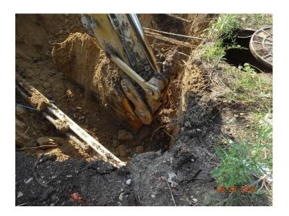
10. Excavating east of MH 2 with two (2) underground fiber optic and one (1) underground electric utility exposed in the northwest corner of the Site.
