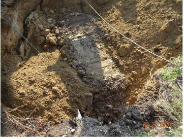
12. Backfilled sanitary sewer trench east of MH 2 with compacted clay.
