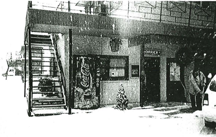
Photograph 1 – Office area of the motel. Note upper balcony. Balcony and roofing material were sampled in this location.
