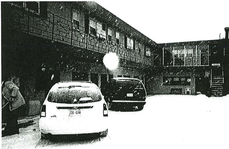
Photograph 2 – Interior courtyard and parking lot for the motel. Former UST's were located near the stairwell to the second floor balcony and rooms.
