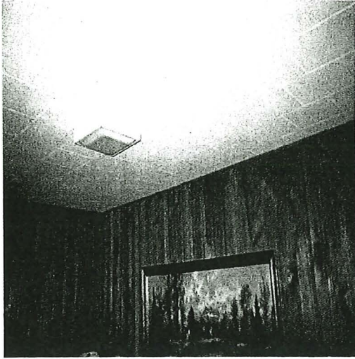
Photograph 10 – Second type of ceiling covering material found in the motel rooms.
