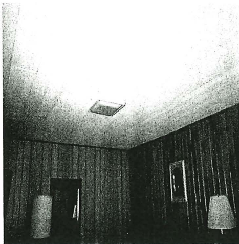
Photograph 9 – One variation of ceiling covering materials found in the motel rooms.
