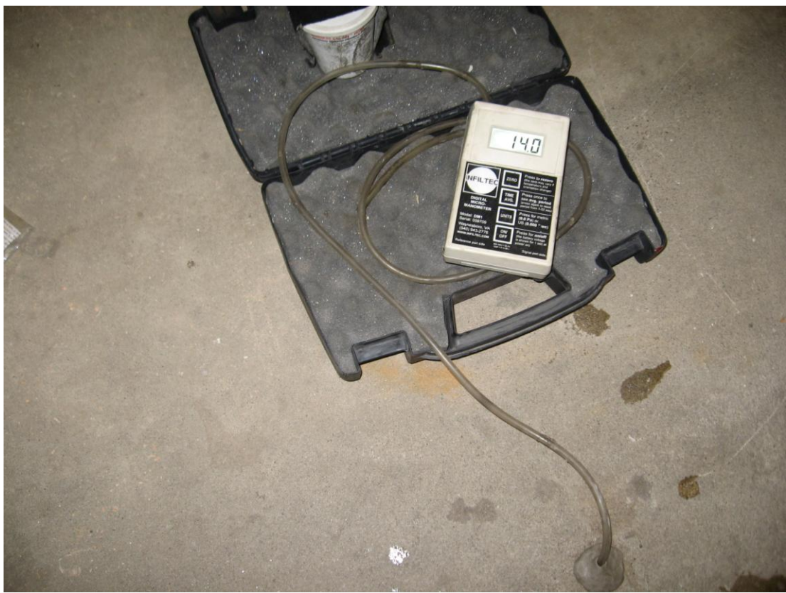
Photograph #: 9 Date: 10/11/2012 Direction: Southern half of site building Subject: Post-installation verification testing
