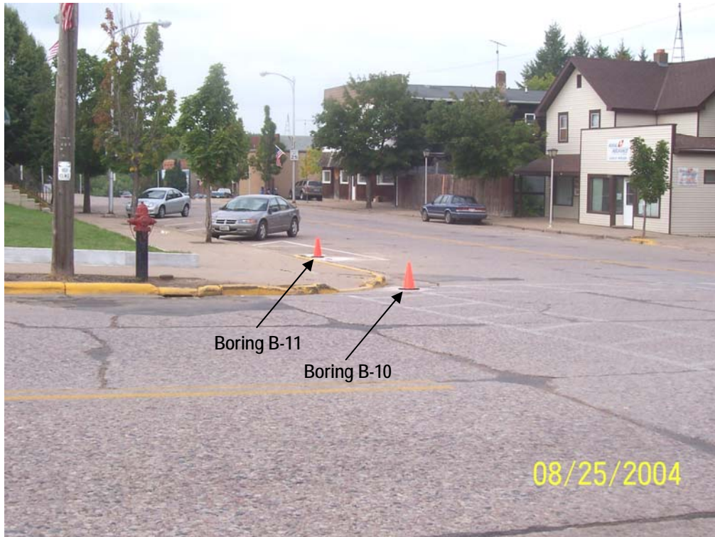
Boring locations looking north.
