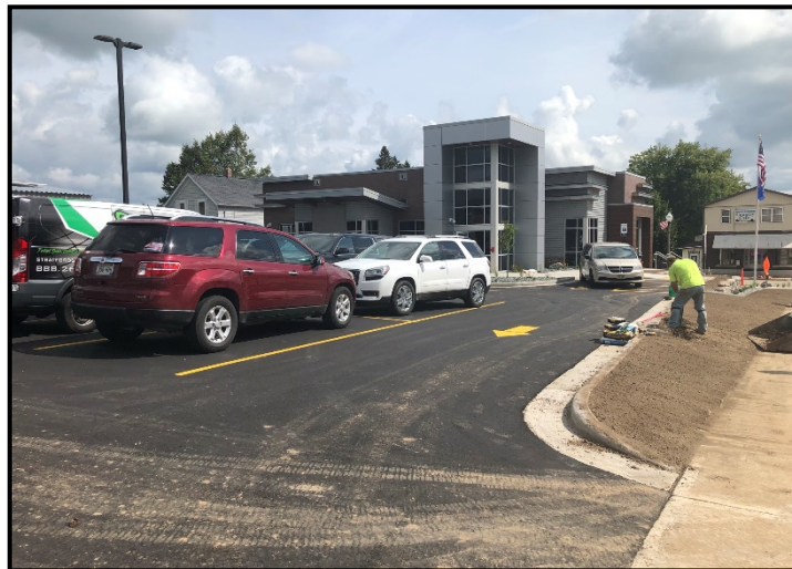
(8-31-2021) Forward Bank - New Construction Complete - View East Along Southern Boundary
