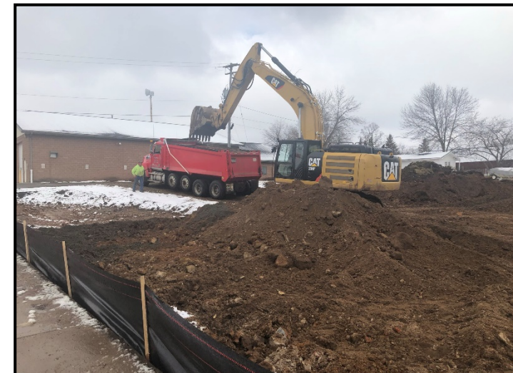
(3-17-2021) Loading out trucks to Lincoln County Landfill
