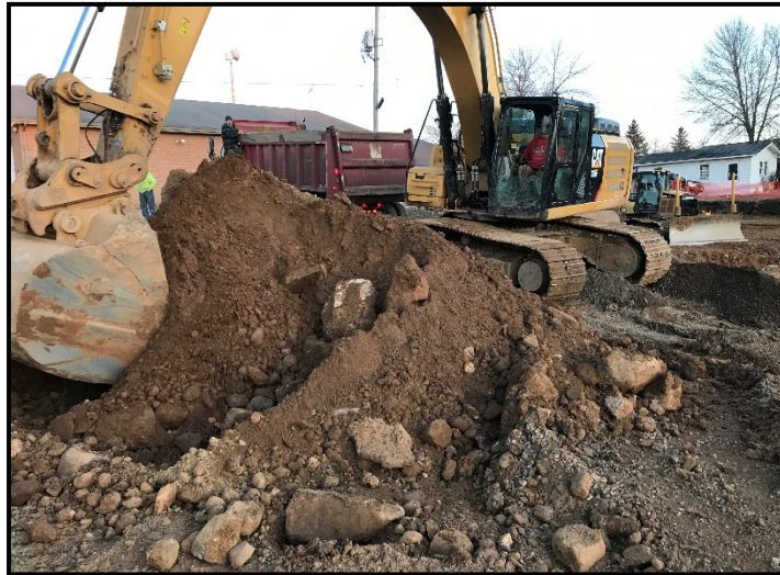
(3-19-2021) Loading Trucks of Contaminated Soil for Landfill Disposal
