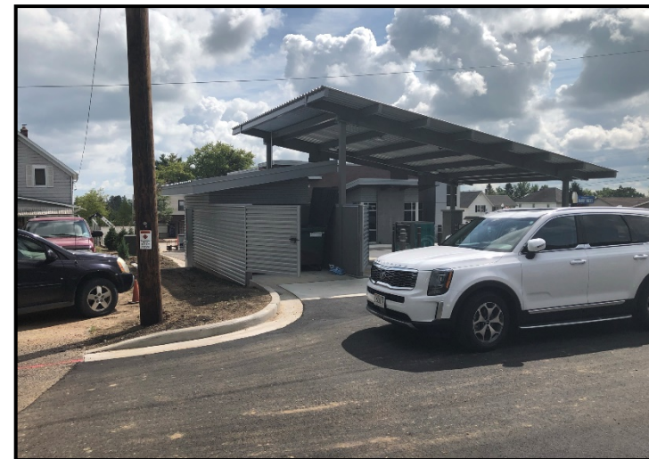
(8-31-2021) Forward Bank - New Construction Complete - View East Along North Boundary
