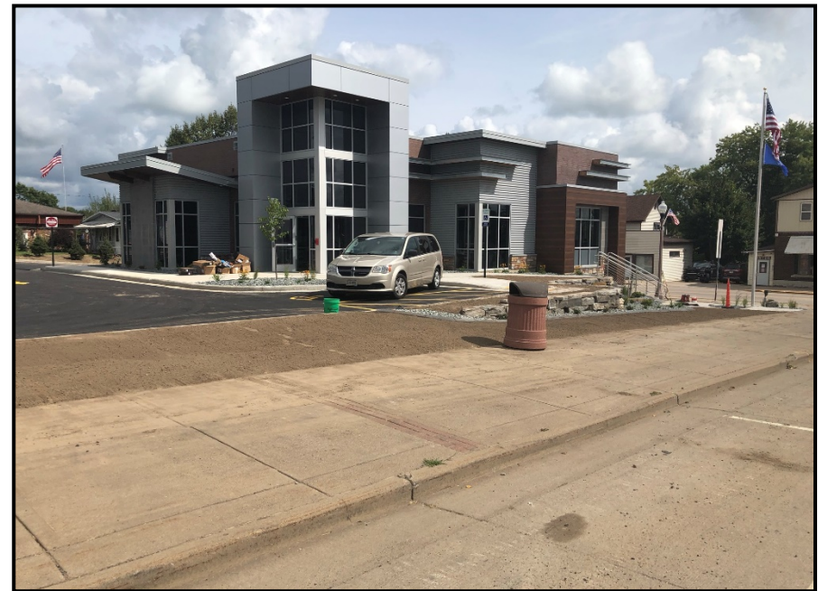
(8-31-2021) View Northeast at New Forward Bank Building
