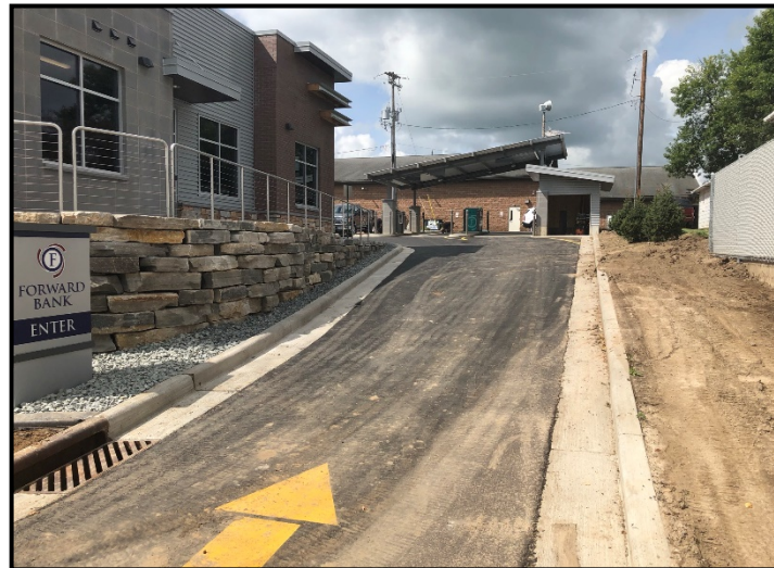
(8-31-2021) View West Along North Boundary
