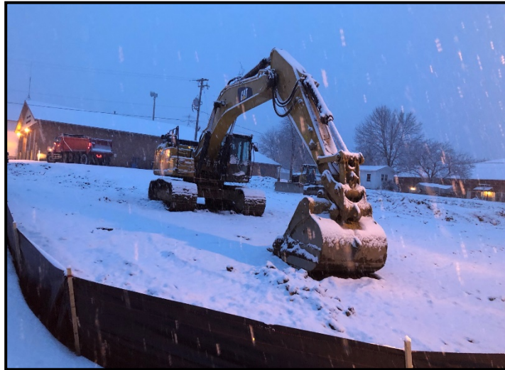
(3-17-2021) Excavating soil in area of historical contamination
