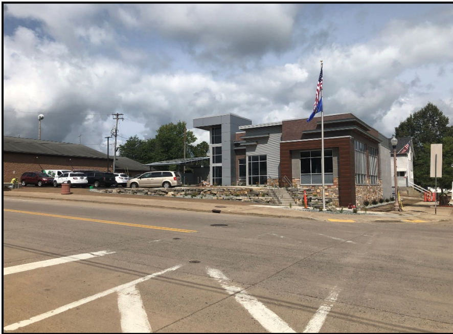
(8-31-2021) View North at New Forward Bank Building
