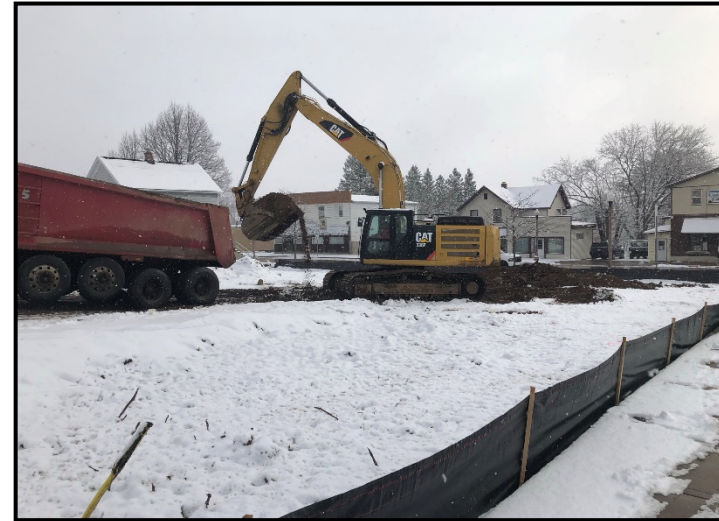
(3-17-2021) Excavating soil in area of historical contamination
