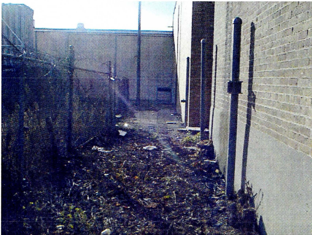
Area Between Valleycast Building and East Fence, Facing South
