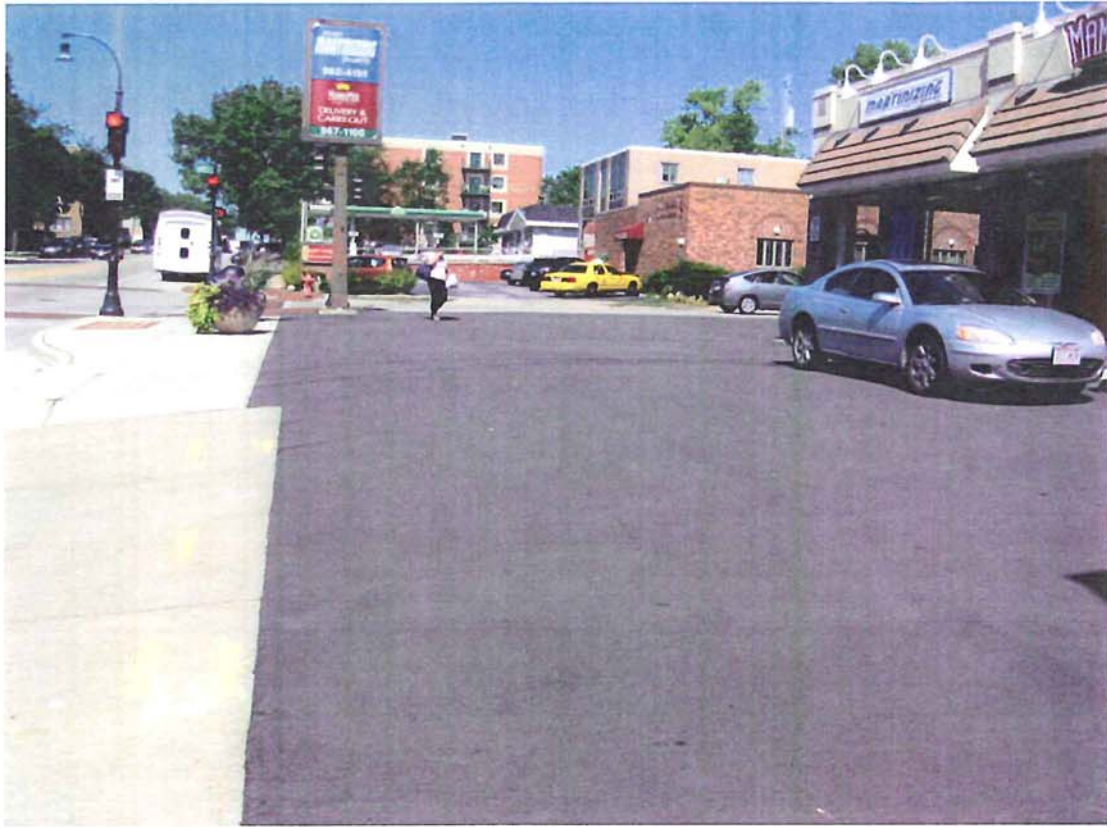
Photograph #: 1 Date: 9/8/2011 Direction: Facing North Subject: Asphalt over excavation area
