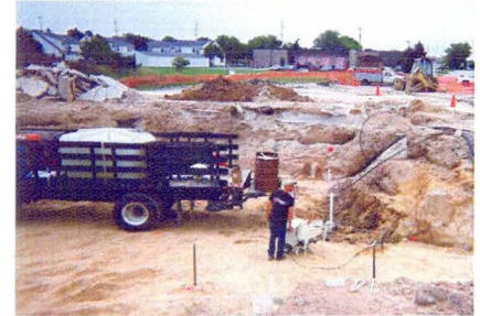
Initial carbon injection within partially backfilled excavation
