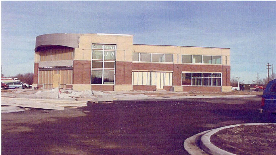
View of Medical Office Building Near Completion of Construction.
