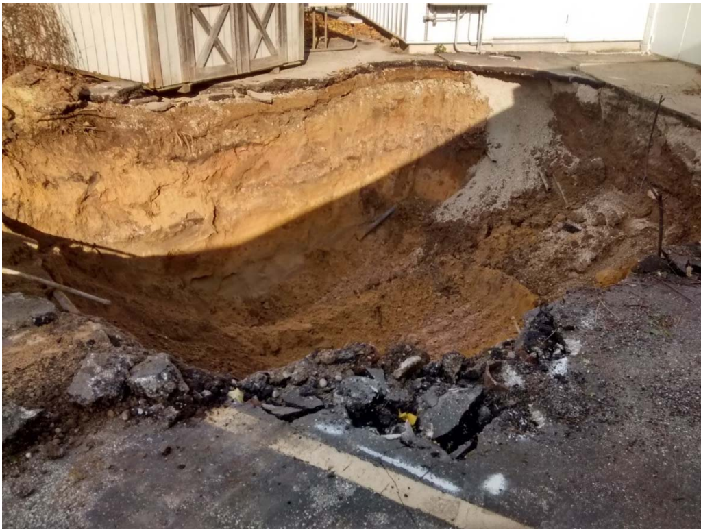
Excavation in progress, facing northwest
