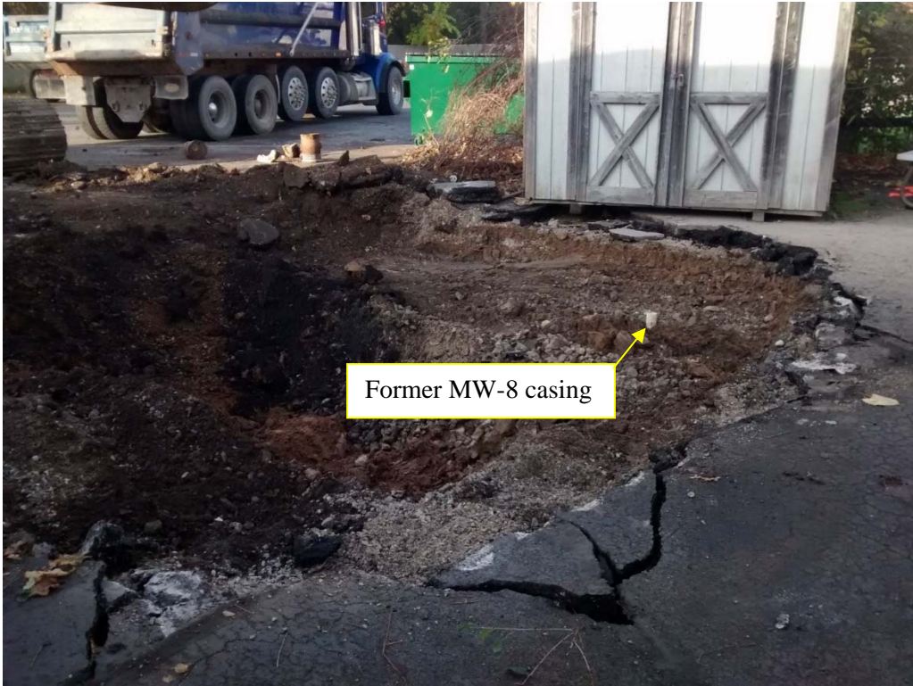
Beginning excavation, facing west
