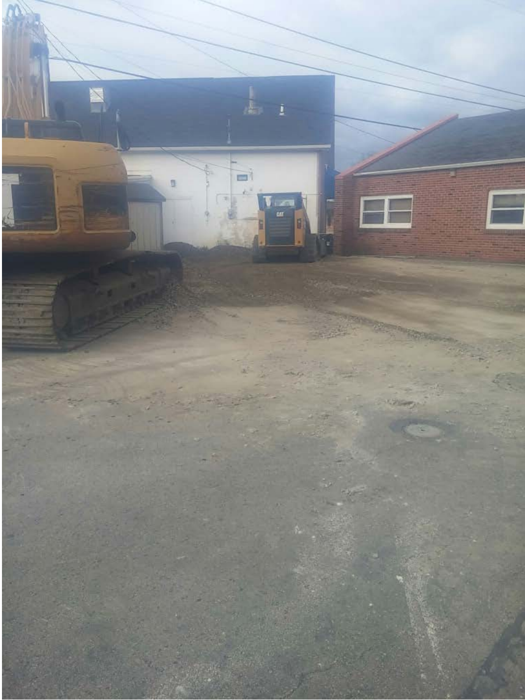
Backfilling complete, facing northeast
