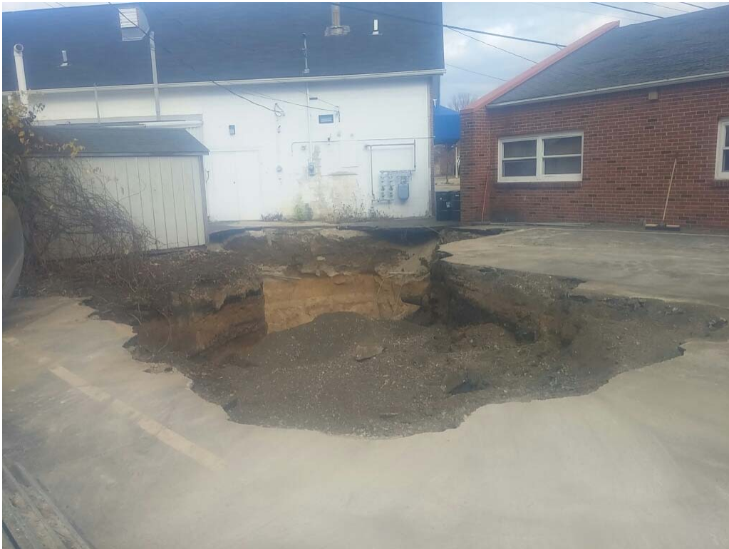
Backfilling in progress, facing northeast
