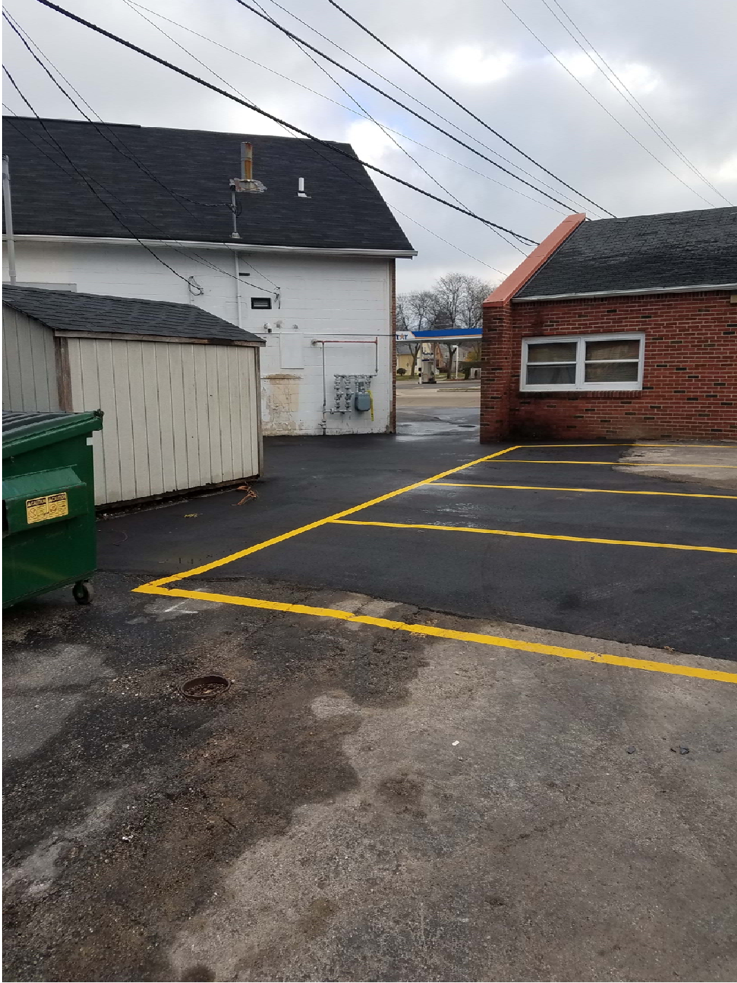
Asphalt repaired and re-striped, facing northeast
