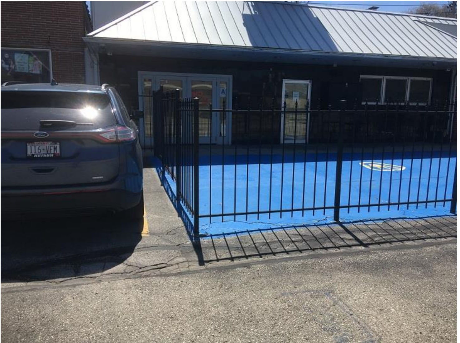
View of the asphalt/concrete cap in the north parking area. View is to the south.
