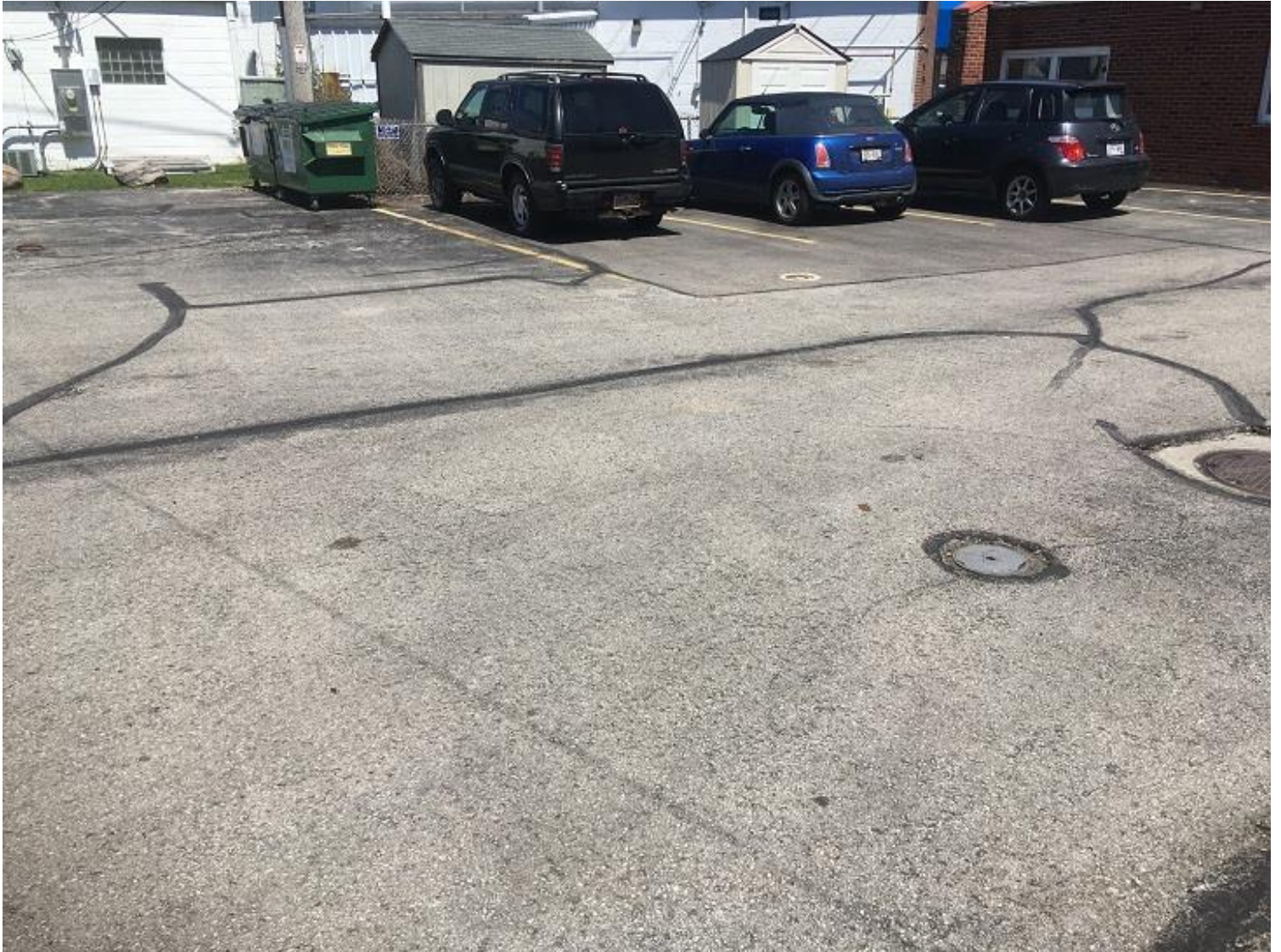
View of the asphalt cap in the south parking area. View is to the northeast.
