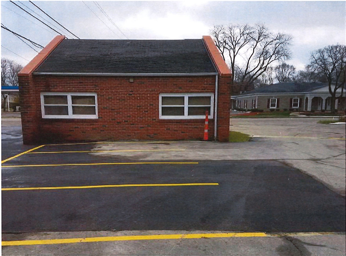
Overview of the asphalt cap and west building foundation, facing east.
