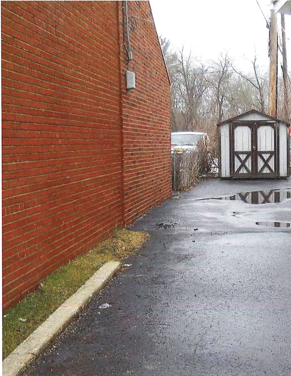
View of the north building foundation, facing west.
