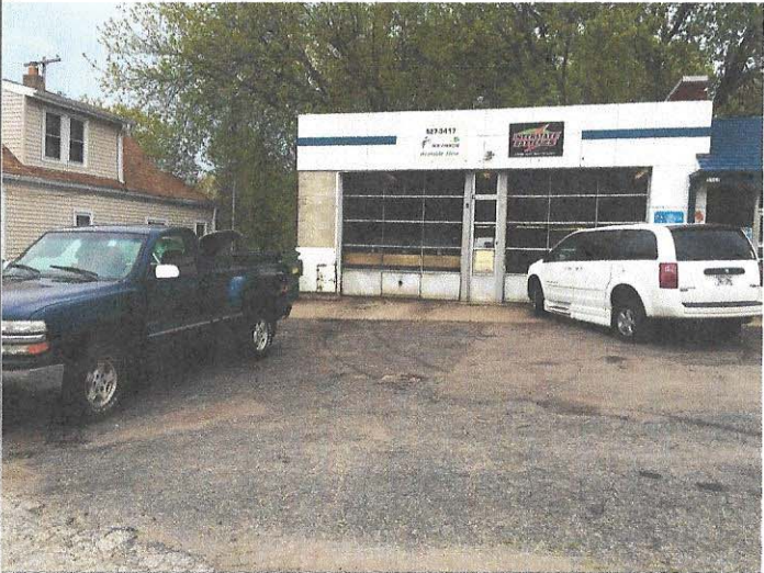
Title: Area of Cap to be Maintained, looking south.
