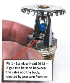
The sprinkler head is located in the southwest corner of Building 69 above a shed (see Pic 3). This is a new fire suppression system that was started up at the beginning of October 2023.
