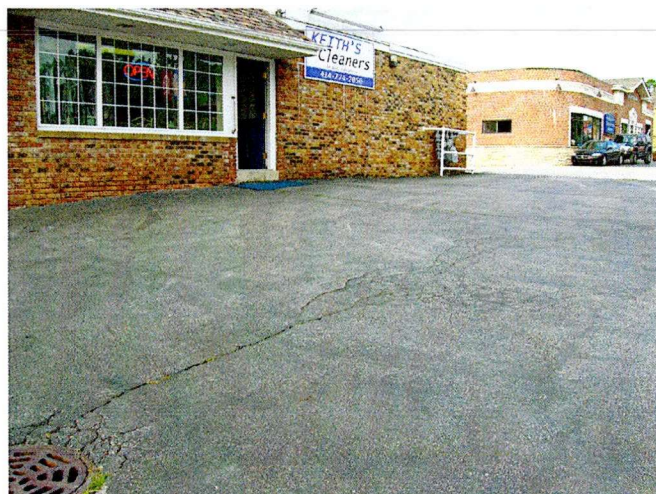
Pavement cover – facing southwest from the northeast corner of the property
