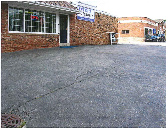
Pavement cover – facing southwest from the northeast corner of the property
