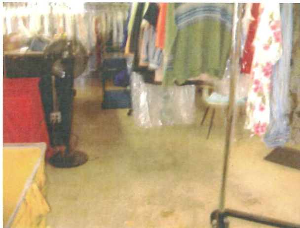
Concrete Floor Condition
