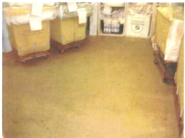
Concrete Floor Condition
