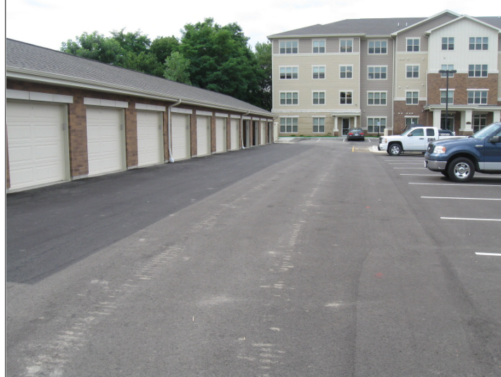
Title: View southerly across pavement near the garage structure.
