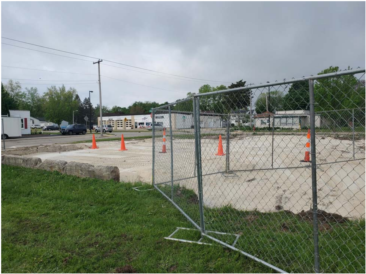
Overview of area showing complete backfill with screening material, facing southwest.
