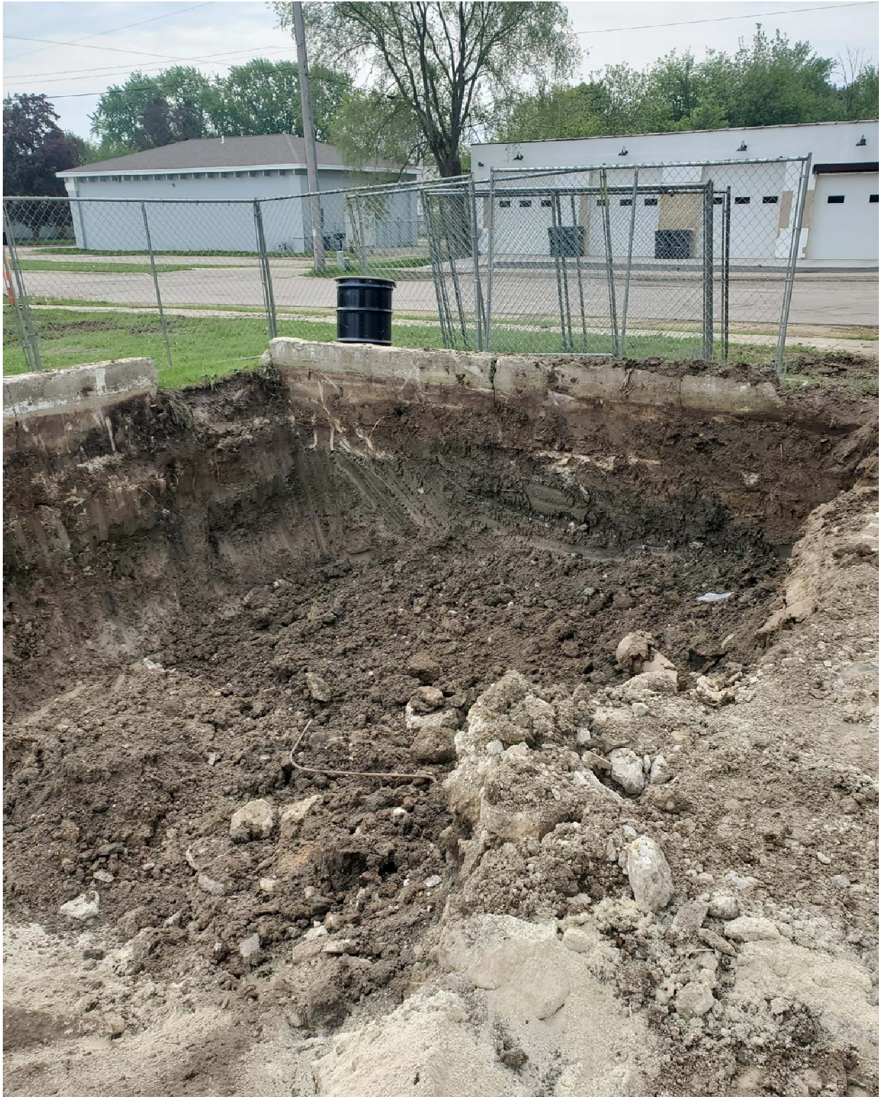
Completed southeast corner of excavation, facing southeast.
