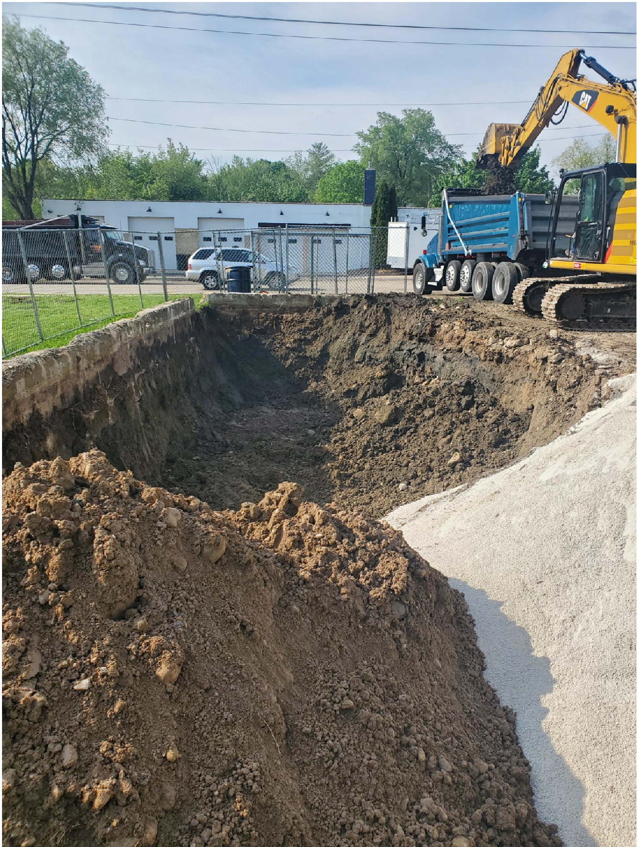
East side of the excavation, facing south.
