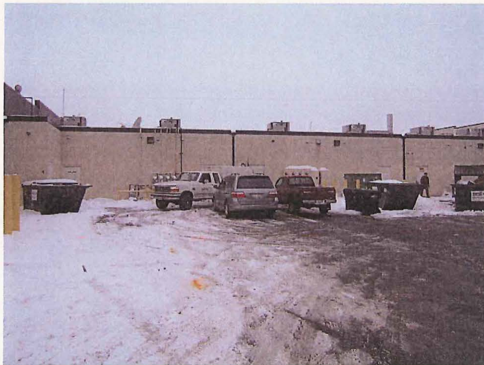
Photo No. 4: Photo showing asphalt pavement behind the dry cleaners tenant space, view to the west; photo taken on December 13, 2005.
