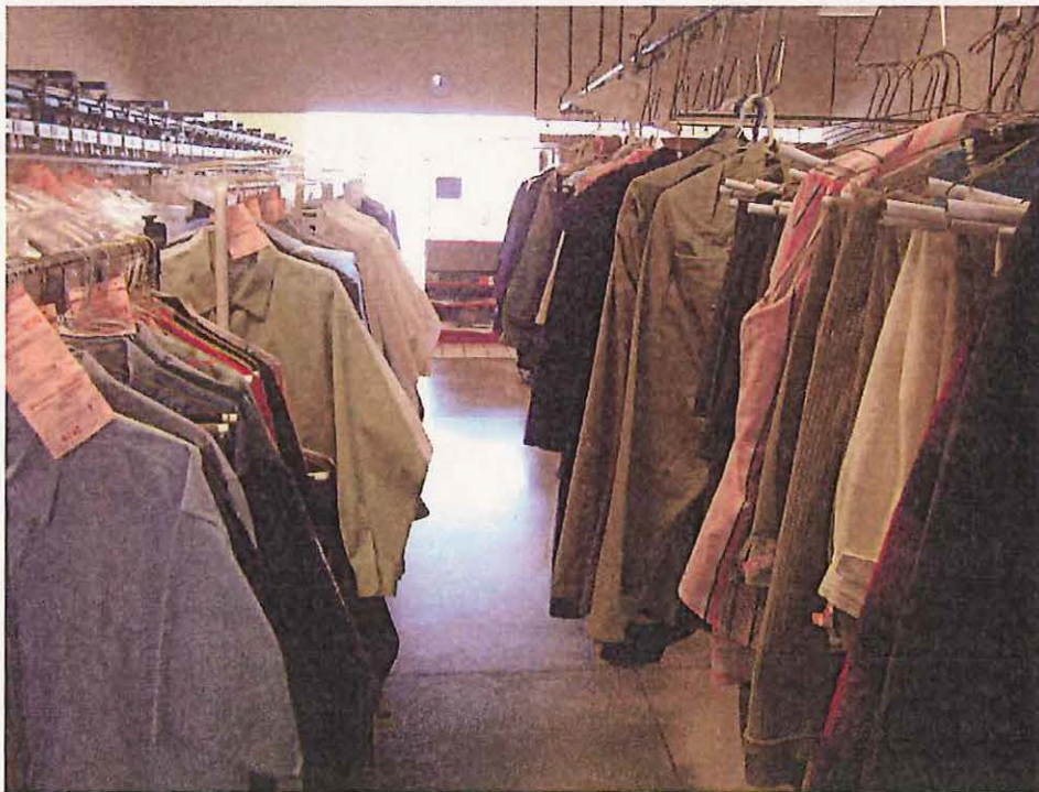
Photo No. 8: Photo showing concrete floor slab inside dry cleaner tenant space; photo taken on February 23, 2006.
