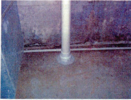
Suction point in the basement below the Scoop
