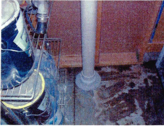
Suction point near dry cleaning equipment
