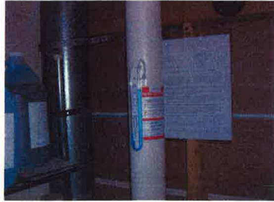
Suction point near dry cleaning equipment
