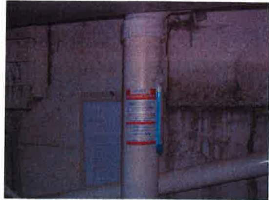
Suction point in the basement below the Scoop
