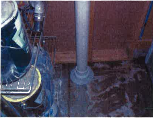
Suction point near dry cleaning equipment
