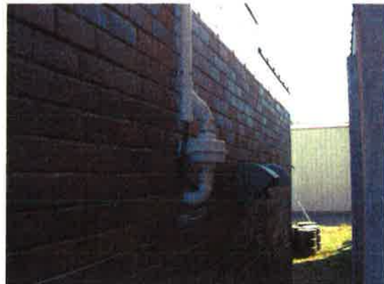
Radonaway GP501 fan for both suction points in laundry area
