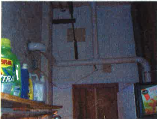
Piping to 2 nd suction point located near Water heater @SE corner
