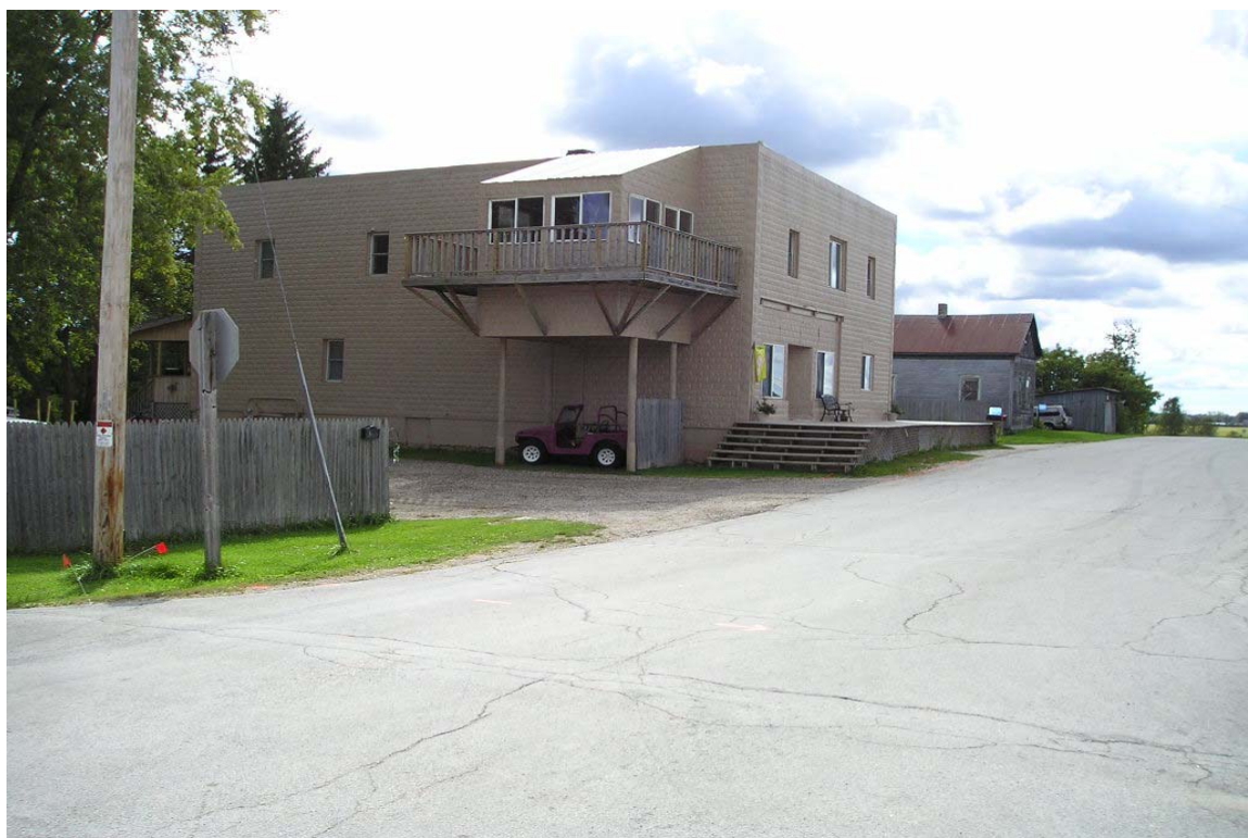
Location of MW-1 (just to right of deck stairs)
