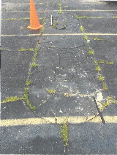
Title: Former pump island - area of asphalt cap.
