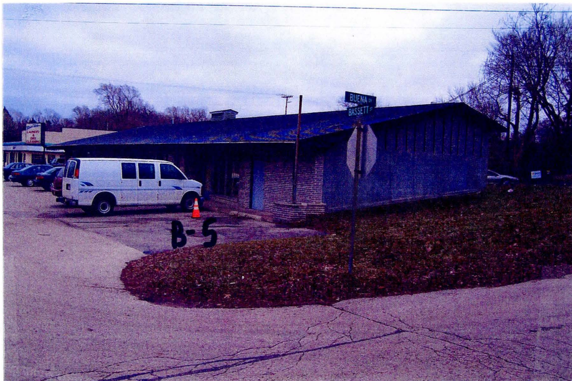
Photo Description: Pictured is the location of boring B-5 on the northwest corner of the lot. Photo Direction: Southeast
