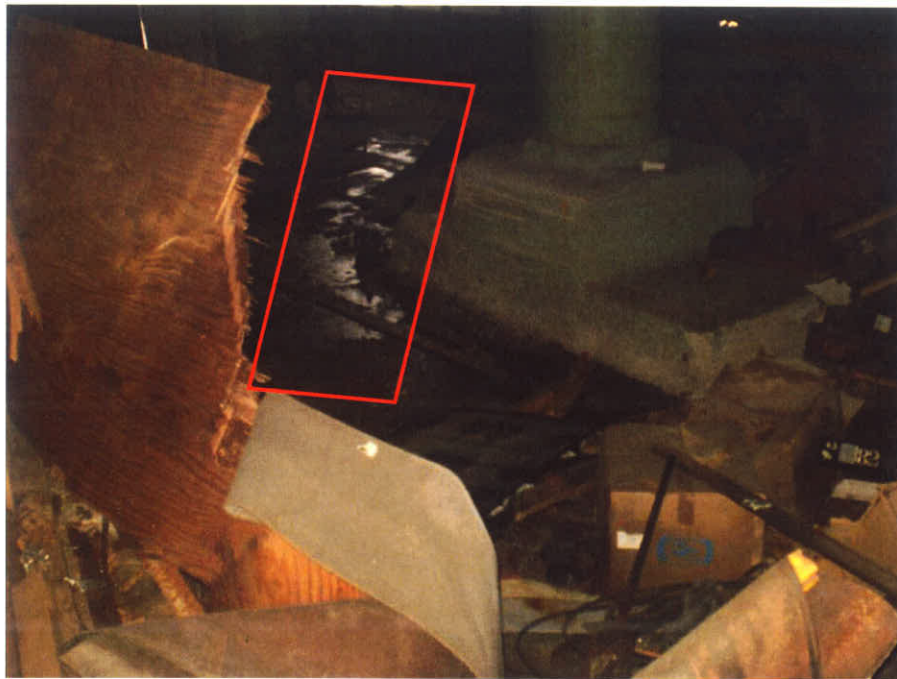
Photograph No.: 1 Photographer: Caitlin Ruza Area: Bldg K-Loading Dock TDD Number: TO-05-10-12-0002 Contract: EP-S5-10-10, OTIE Date: January 24, 2011 Site Name & Location: Mirro-Spirtas Site, Manitowoc, Manitowoc County, Wisconsin Photograph Subject: Dumped material and oil sheen leading to the drain inside the loading dock in Building K
