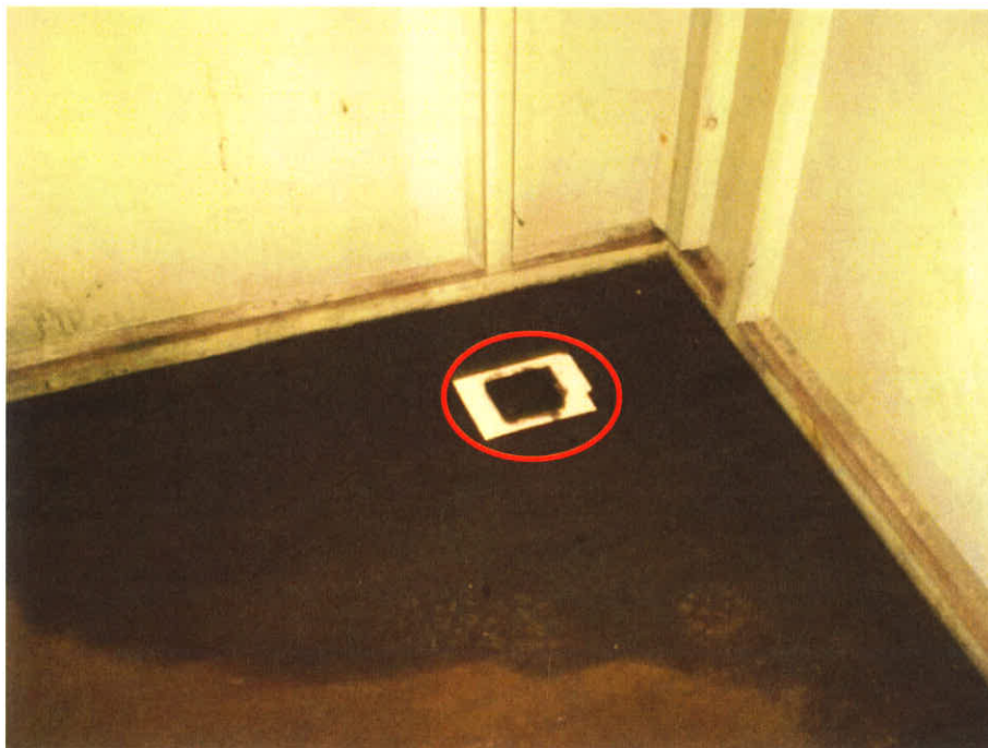
Photograph No.: 6 Photographer: Caitlin Ruza Area: Building I-Transformer TDD Number: TO-05-10-12-0002 Contract: EP-S5-10-10, OTIE Date: January 24, 2011 Site Name & Location: Mirro-Spirtas Site, Manitowoc, Manitowoc County, Wisconsin Photograph Subject: MS-WP-1 collected from stained area of small room adjacent to the transformer room in Building I (template area shown)
