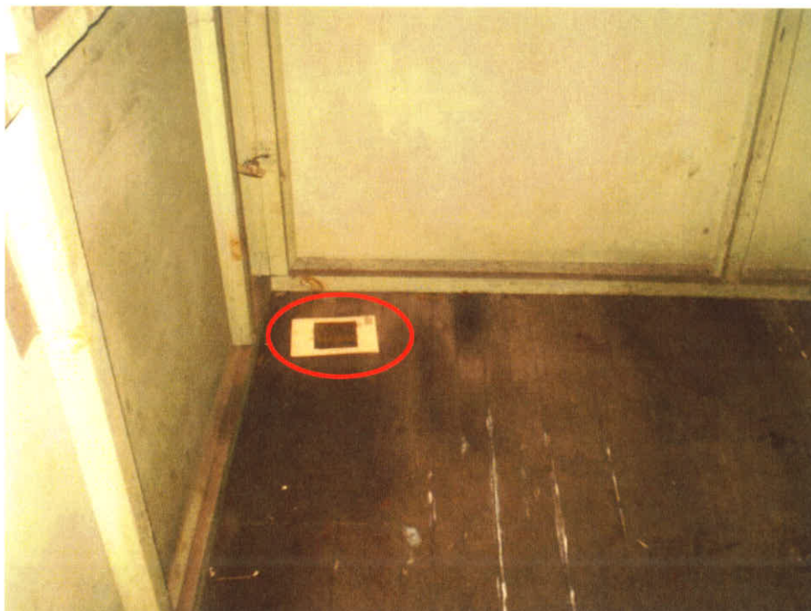
Photograph No.: 7 Photographer: Caitlin Ruza Area: Building I-Transformer TDD Number: TO-05-10-12-0002 Contract: EP-S5-10-10, OTIE Date: January 24, 2011 Site Name & Location: Mirro-Spirtas Site, Manitowoc, Manitowoc County, Wisconsin Photograph Subject: MS-WP-2 collected from unstained area of small room adjacent to the transformer room in Building I (template area shown)
