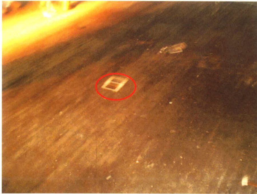
Photograph No.: 9 Photographer: Caitlin Ruza Area: Building I-Transformer TDD Number: TO-05-10-12-0002 Contract: EP-S5-10-10, OTIE Date: January 24, 2011 Site Name & Location: Mirro-Spirtas Site, Manitowoc, Manitowoc County, Wisconsin Photograph Subject: MS-WP-4 collected from edge of saturation staining on flooring outside of the transformer room in Building I (template area shown)
