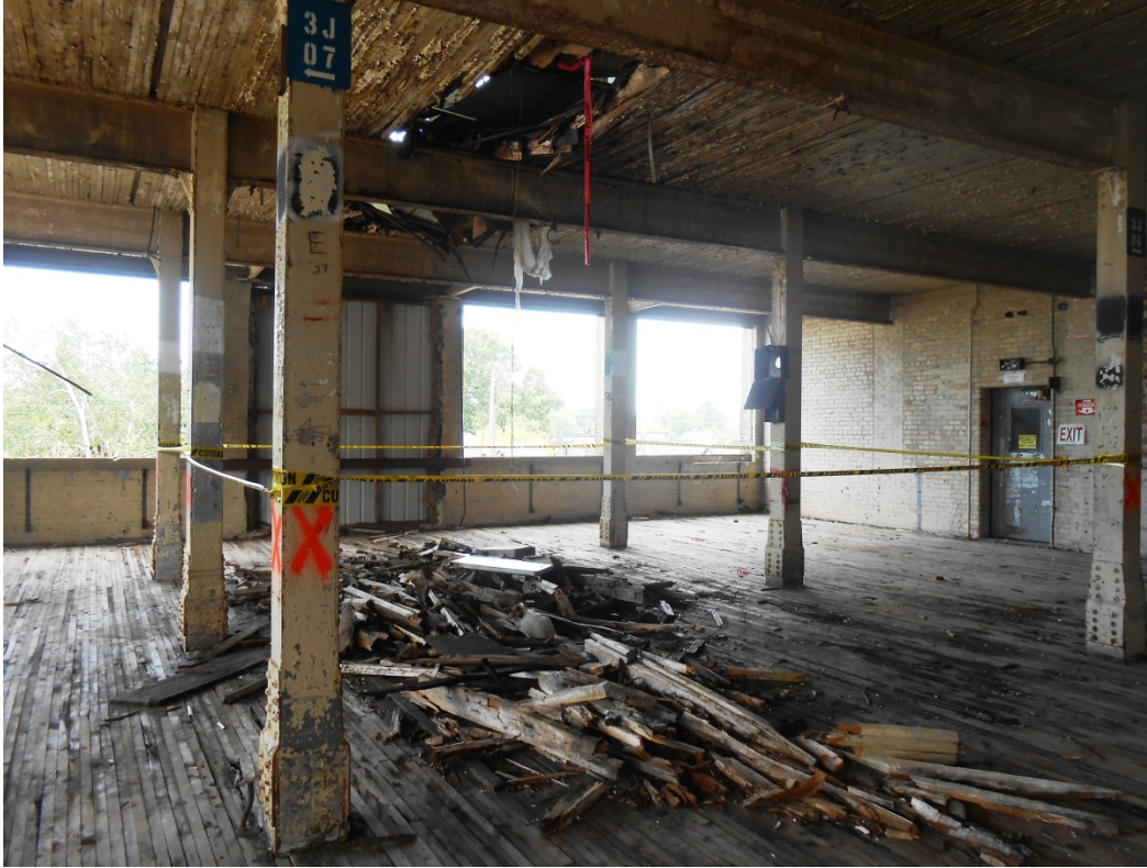
Photo No. 5 – Typical Restricted Area Temporary Barrier
