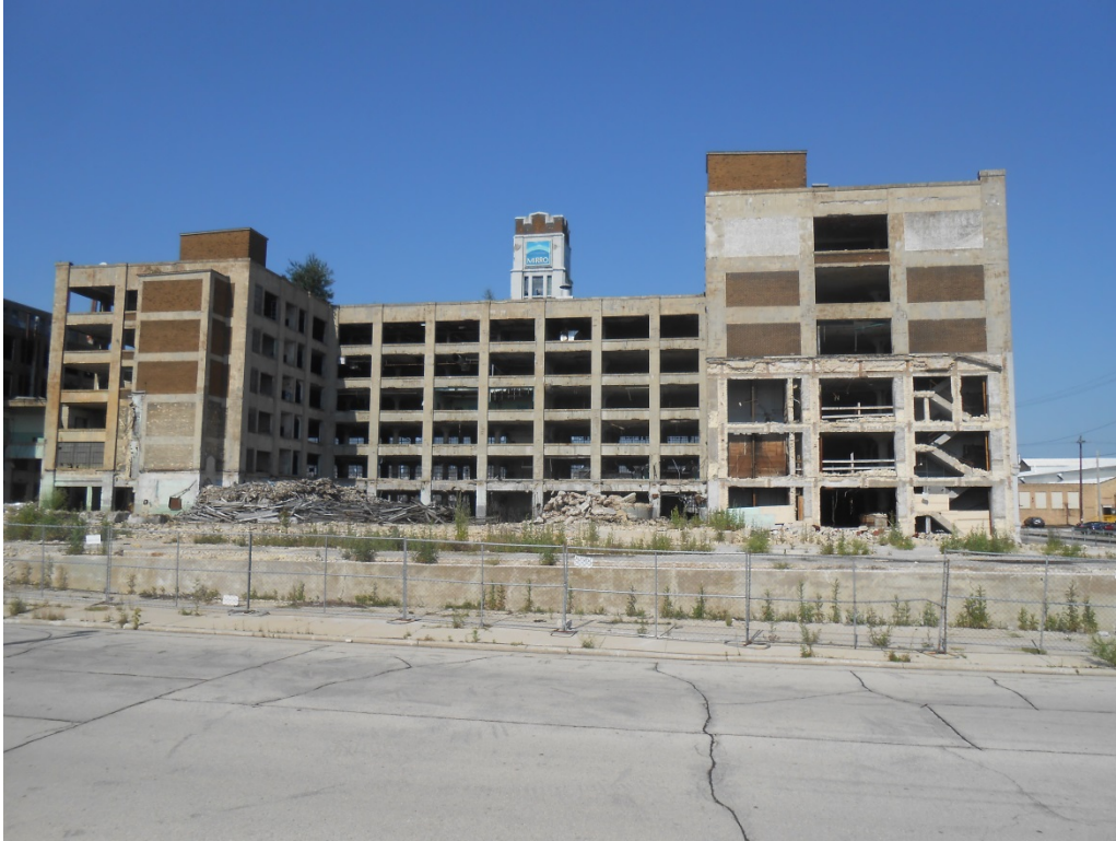
Photo No. 7 – North Building
