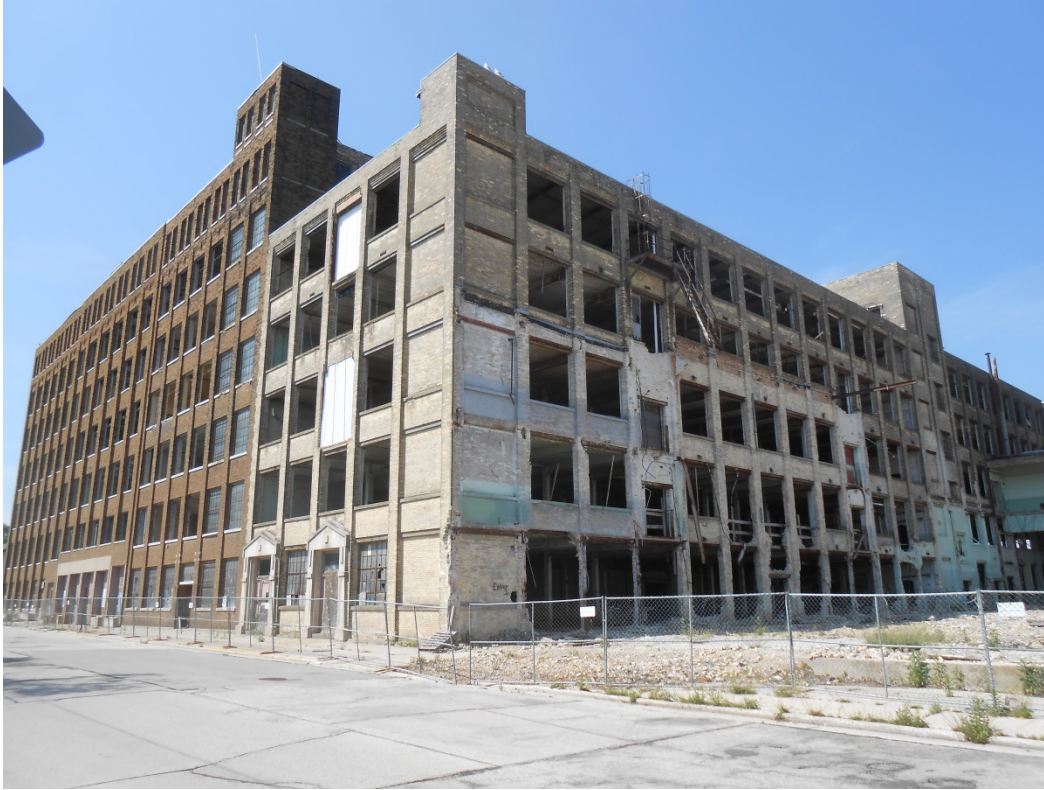
Photo No. 1 – View of South Building
