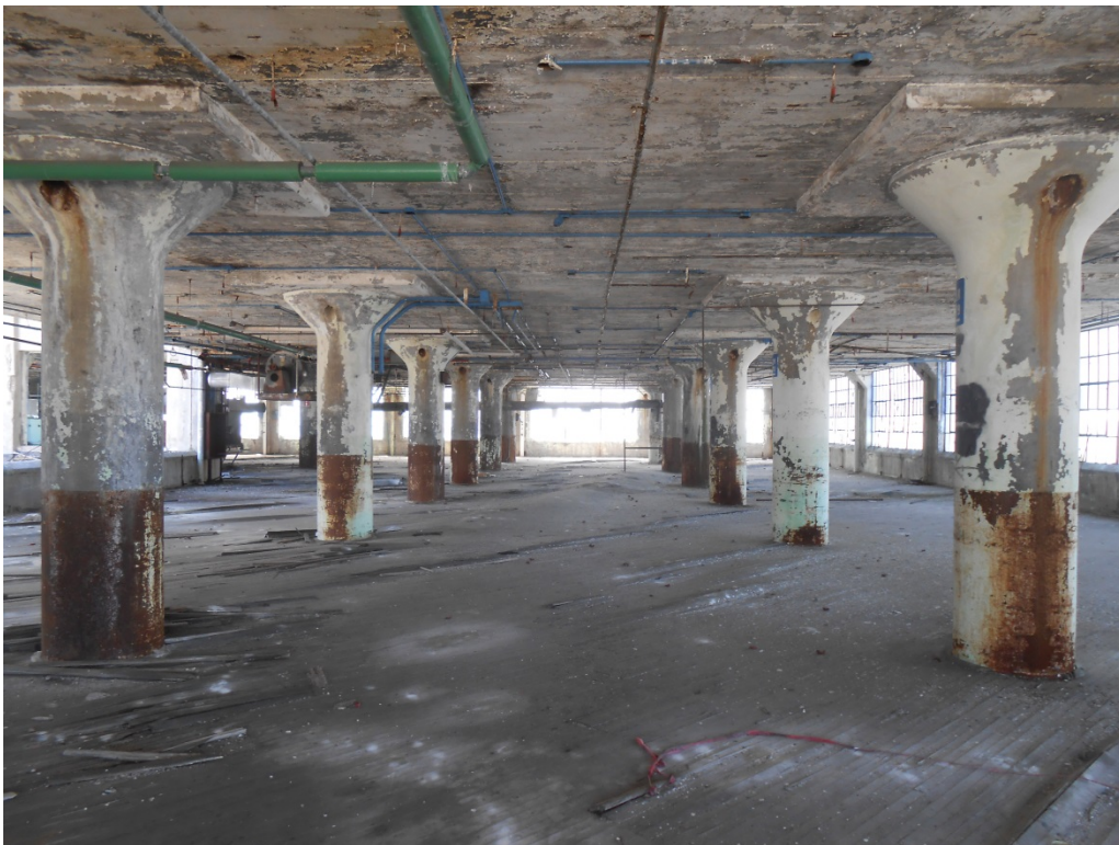
Photo No. 8 – Typical View of Structural System
