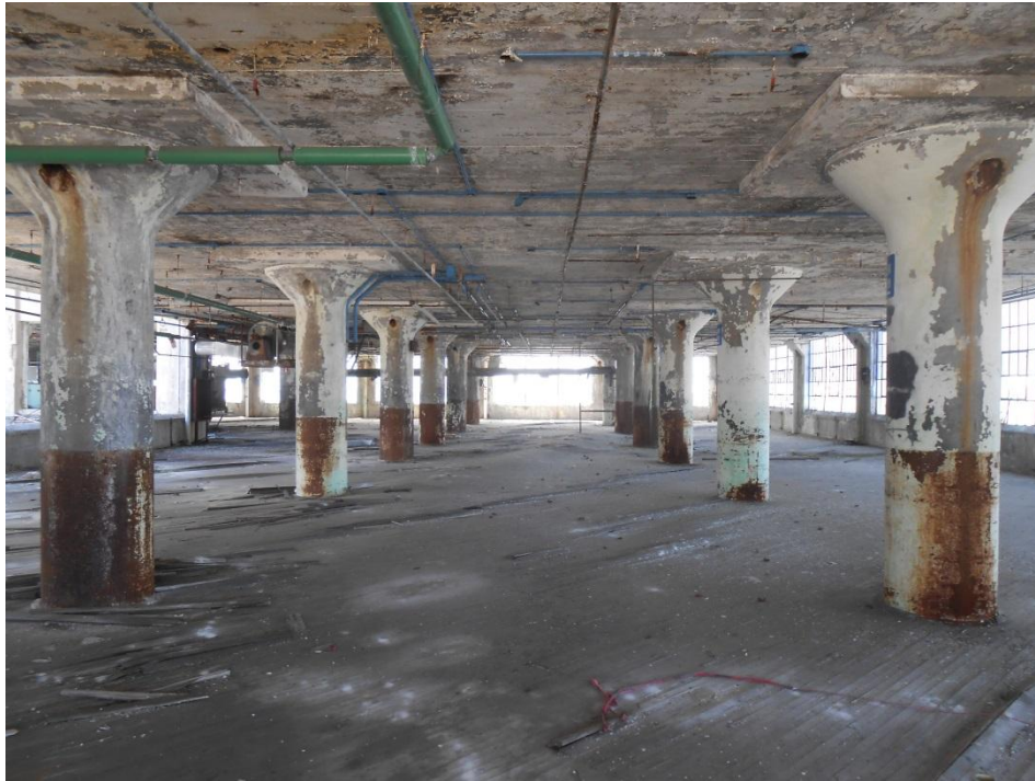
Photo No. 11 – North Building: Cast-In-Place Concrete Columns and Floor Slabs
