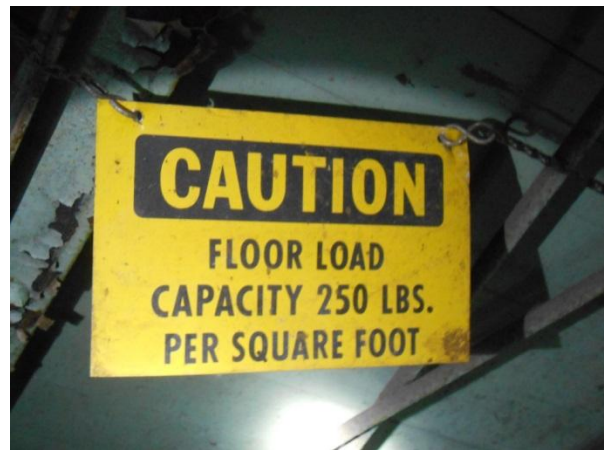
Photo No. 3.1-1: Floor Load Posting
