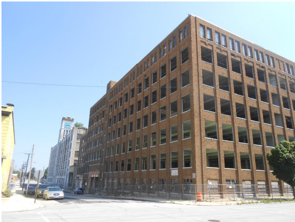
Photo No. 2 – South Building: View Looking Northwest
