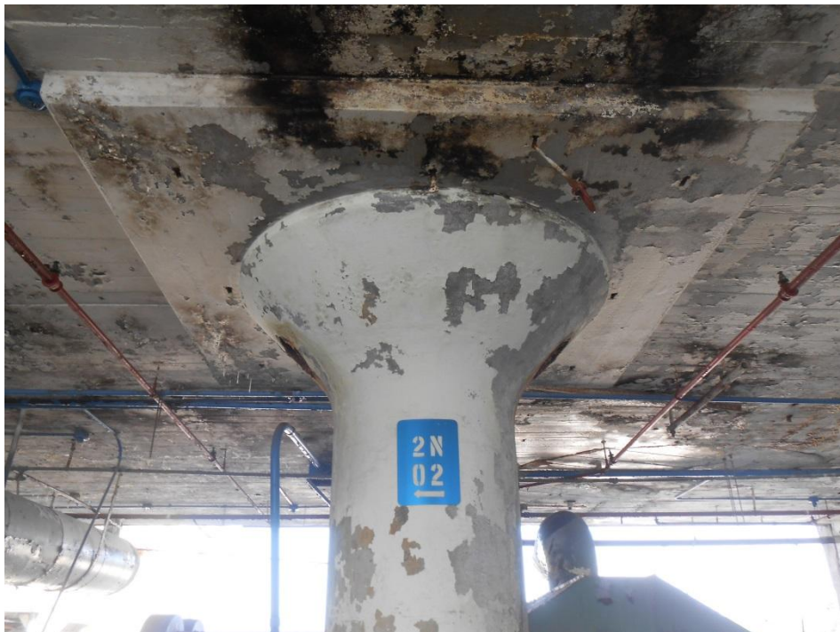
Photo No. 12 – North Building: Cast-In-Place Concrete Column Capital and Drop Panel
