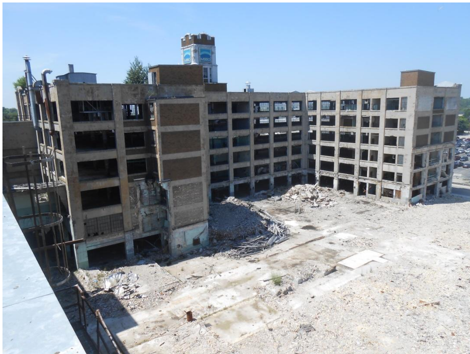
Photo No. 10 – North Building, View Looking Northwest
