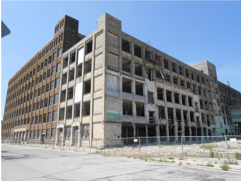
Photo No. 1 – South Building: View Looking Southwest
