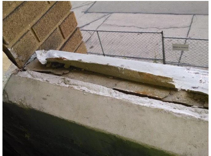
Photo 17: Gray Fiberglass Window Sill Wrap (south building)
