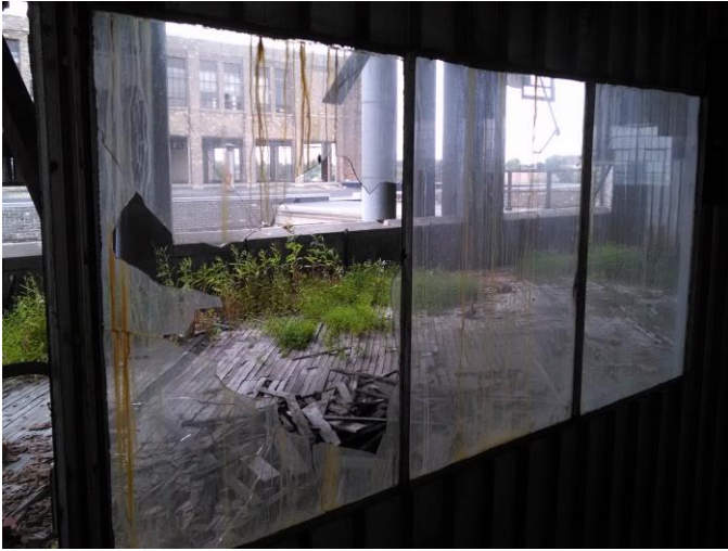
Photo 19: Black Window Glazing
