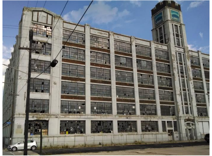
Photo 4: Exterior (west, north)
