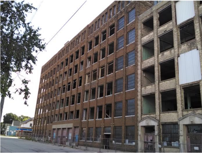
Photo 1: Exterior (east, south)
