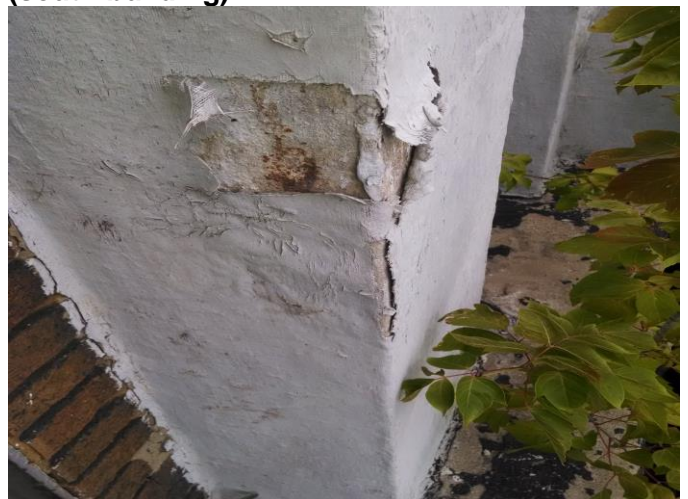
Photo 18: Gray Fiberglass Window Sill Wrap (north building, tower)
