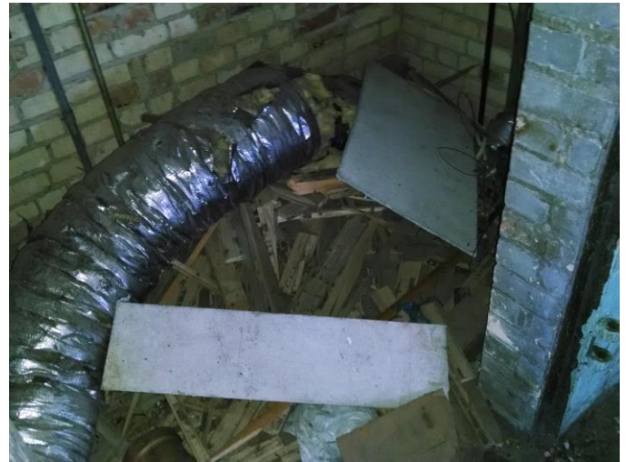
Photo 23: White Ceiling Board / White Panel
