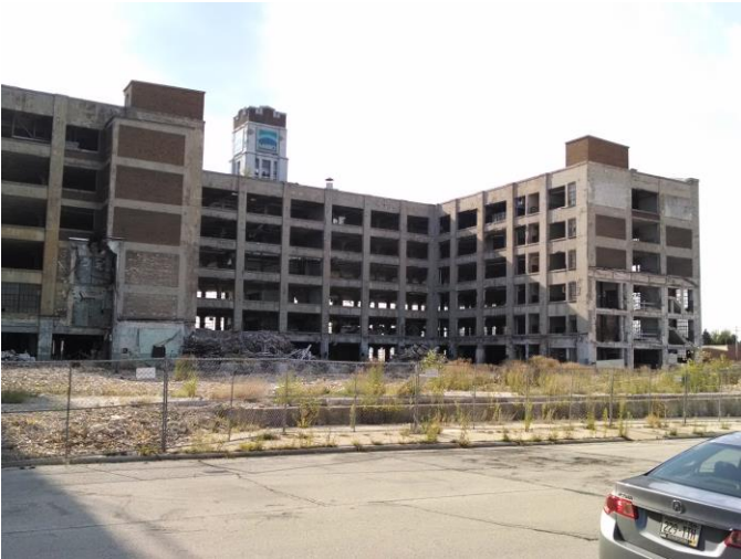
Photo 2: Exterior (east, north)
