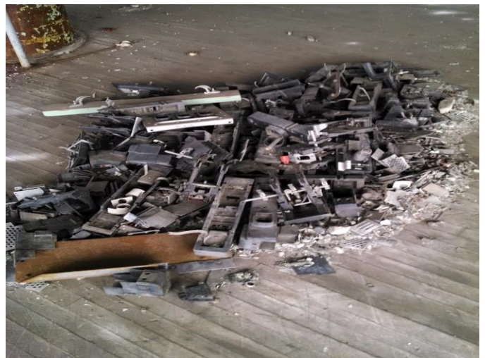
Photo 30: Electrical Isolators (debris pile)
