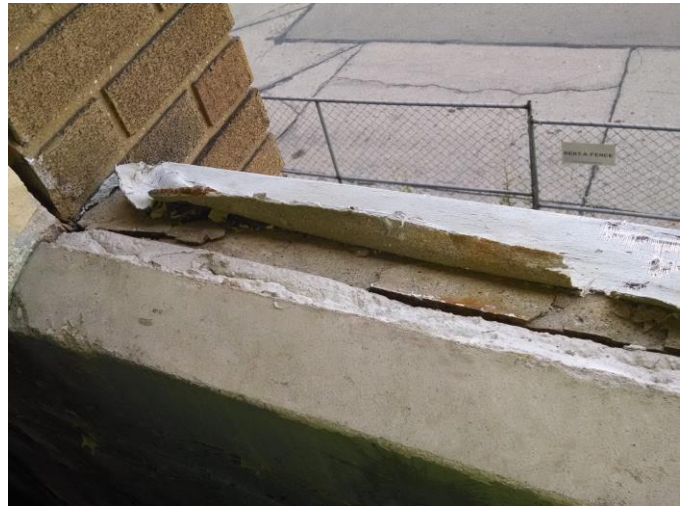
Photo 17: Gray Fiberglass Window Sill Wrap (south building)
