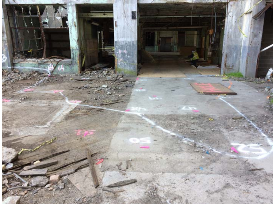
Ground level view of borings, View S
