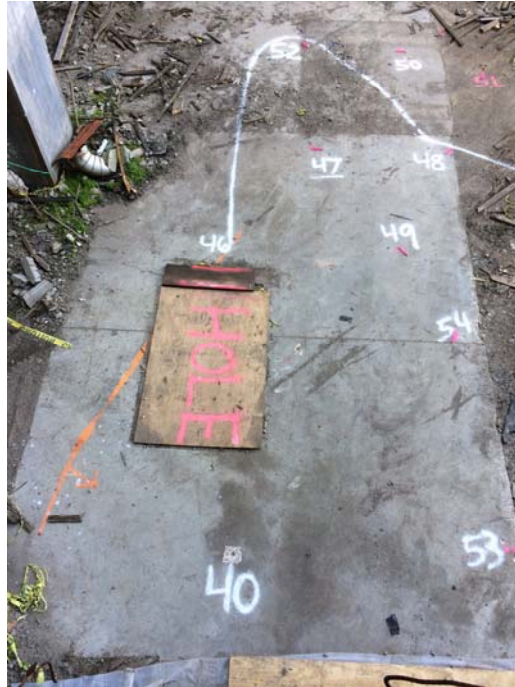
Aerial view of delineation borings, looking down from the 2 nd Story, looking North
