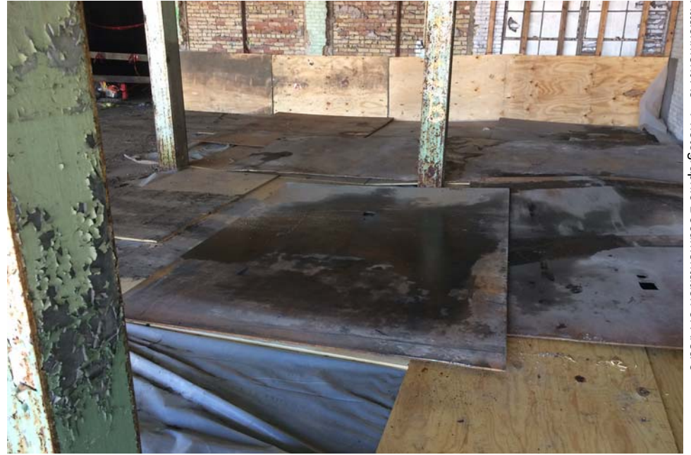
#13 - Installation of temporary cover in Area 8
