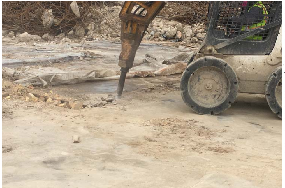
#21 - Breaking concrete around Area 8
