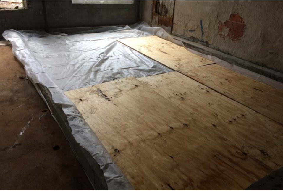
#3 - Temporary cover over former transformer pad in Area 14
