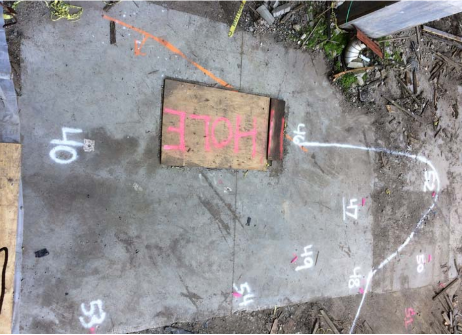
#7 - Delineation of concrete removal area in the Loading Dock
