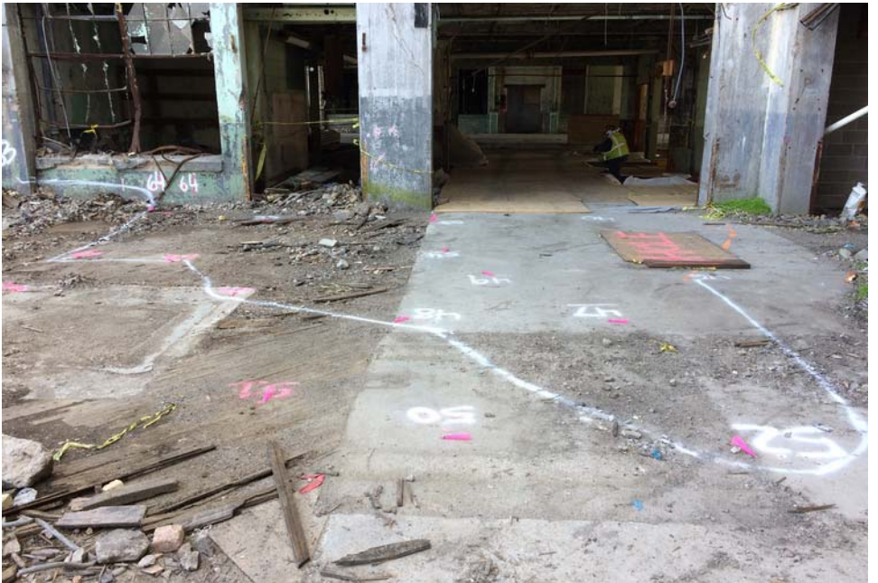
#6 - Delineation of concrete removal area in the Loading Dock
