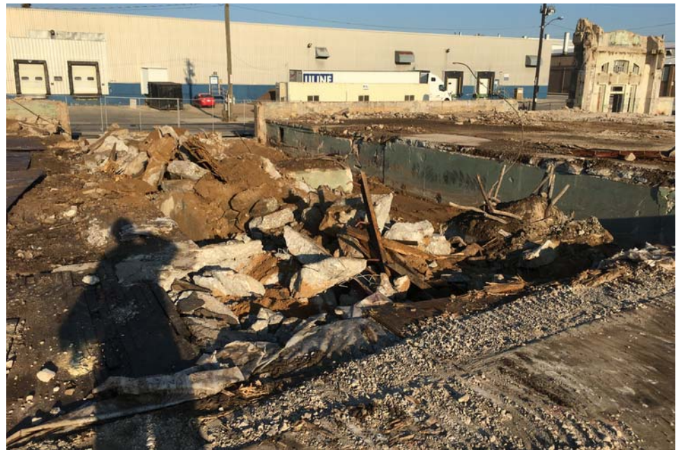
#18 - Demolition of driving apron
