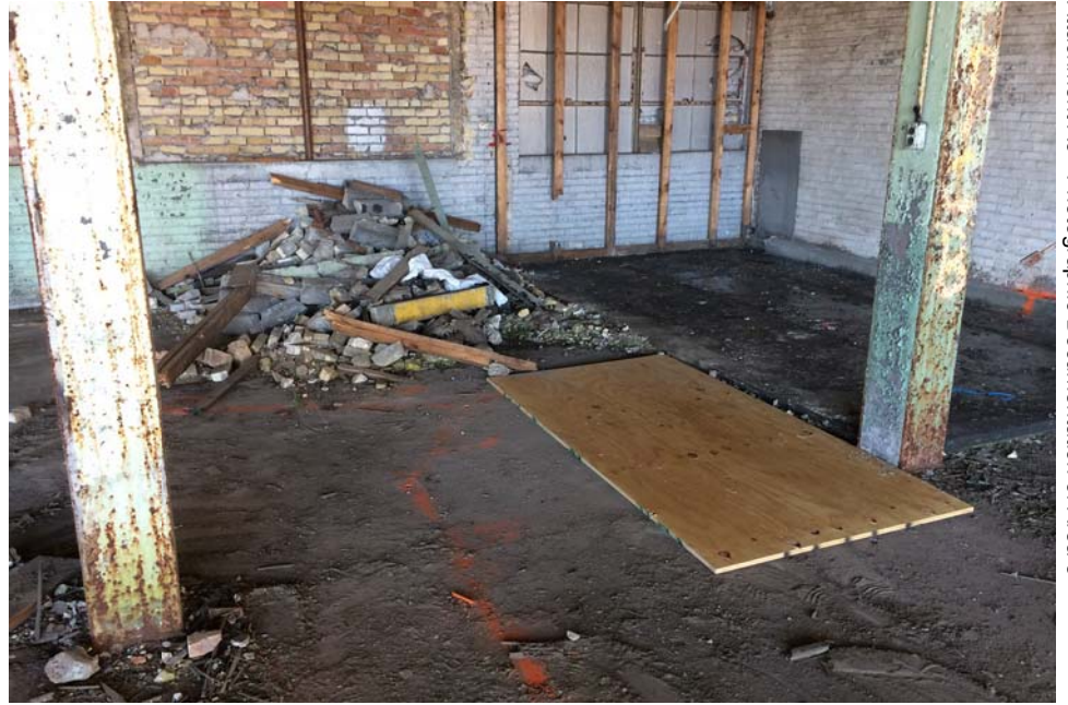
#1 - Area 8 prior to removal
