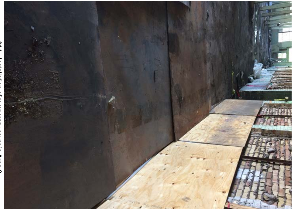
#14 - Installation of temporary cover in Area 8
