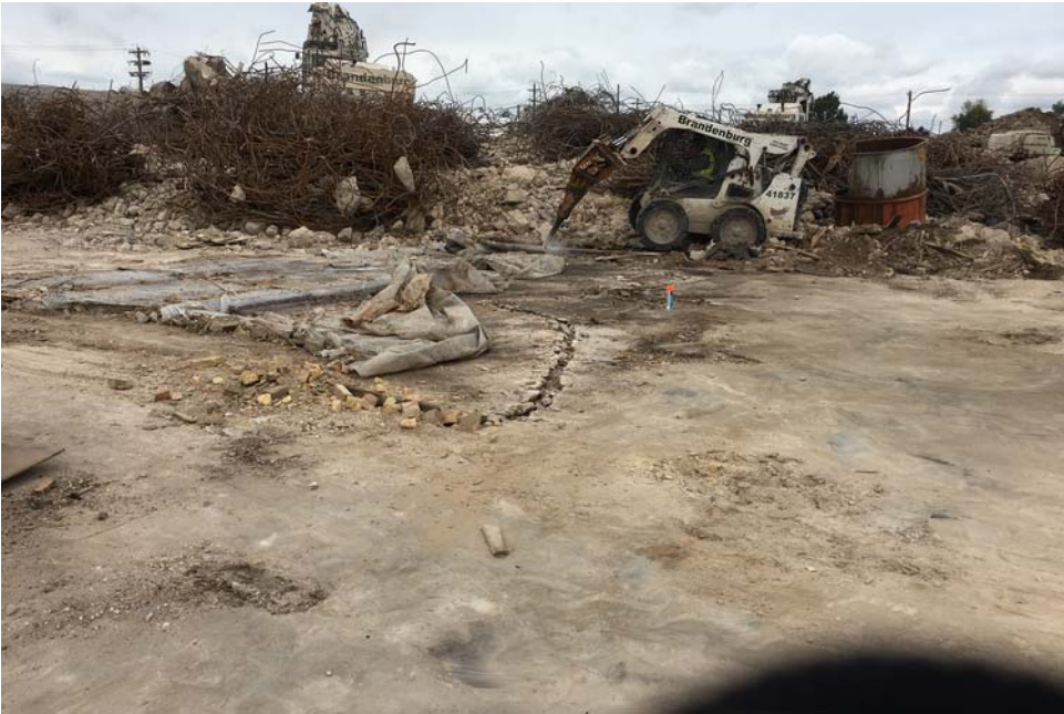
#23 - Breaking concrete from Area 8
