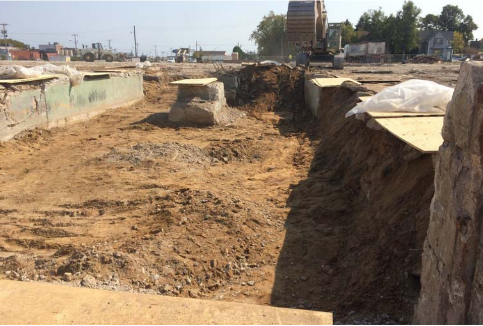
#23 - Driving apron and loading dock lifts after demolition
