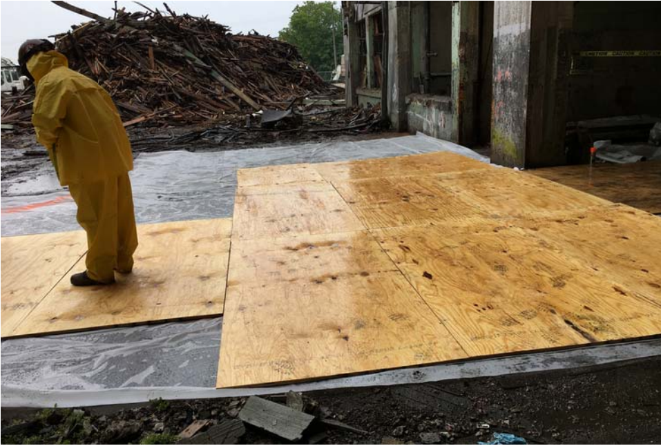
#11 - Temporary cover installed in the Loading Dock
