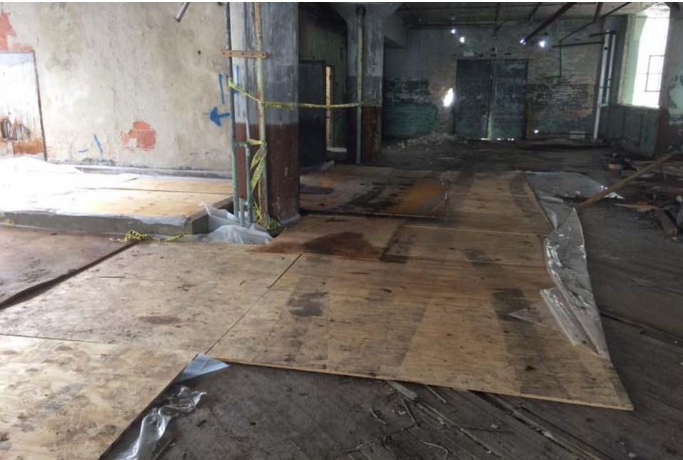
#4 - Temporary cover following transformer removal
