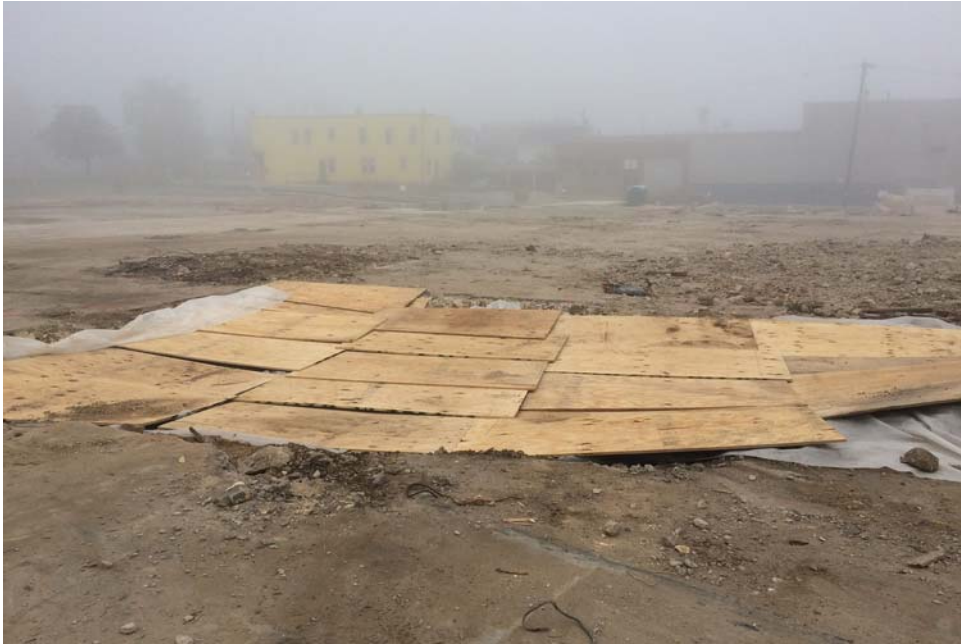
#25 - Area 8 following concrete removal
