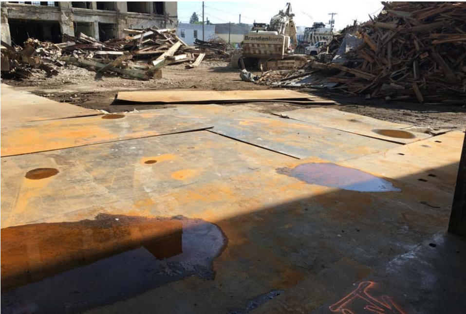
#12 - Temporary cover (steel plates over plywood) installed in the Loading Dock
