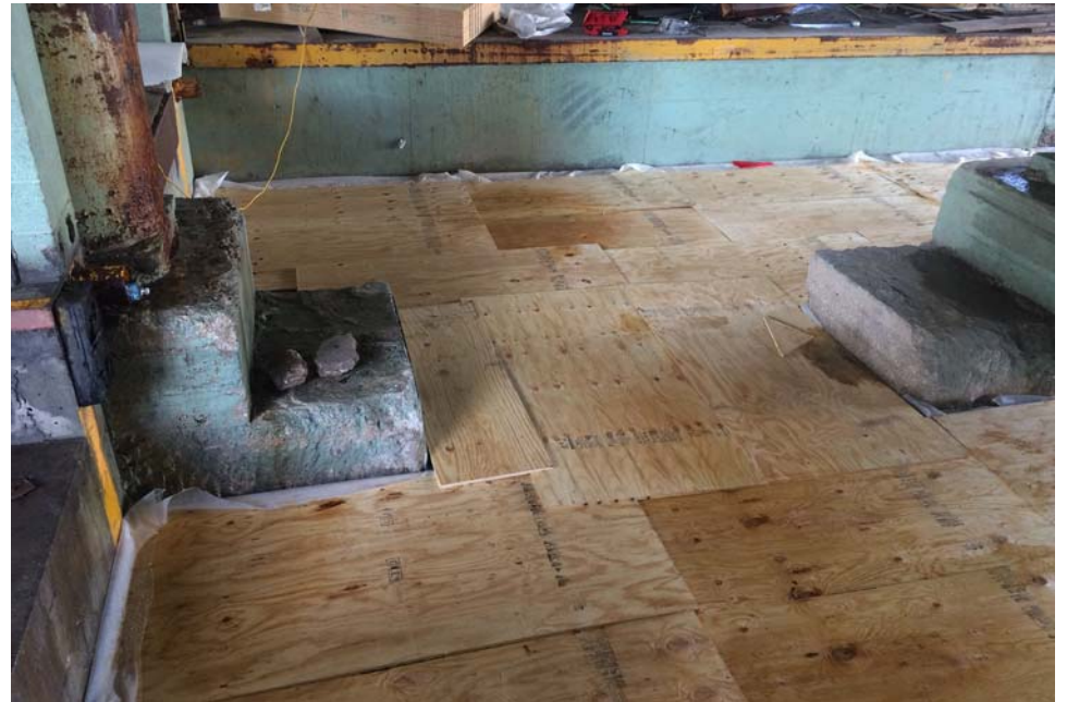
#10 - Temporary cover installed in the Loading Dock
