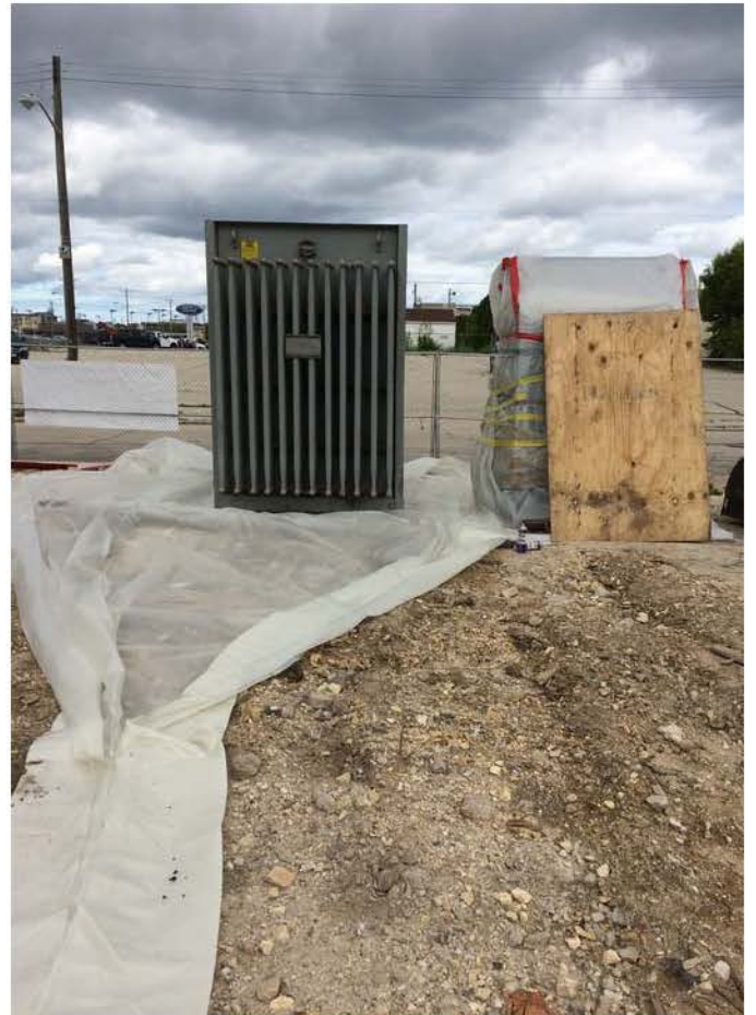
#4 - Transformers being prepared for shipment offsite
