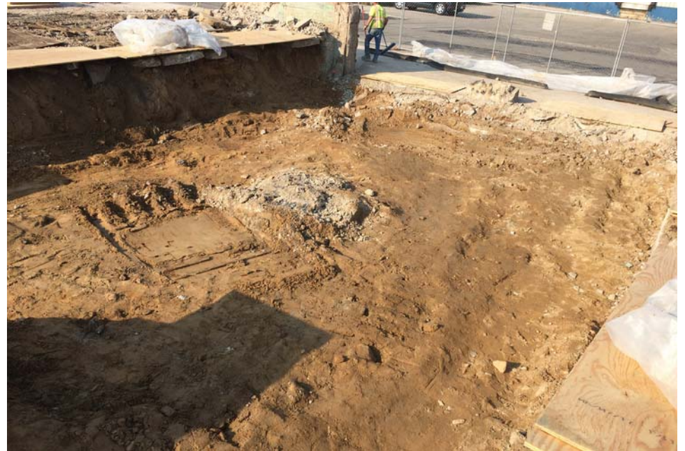
#22 - Driving apron following concrete removal
