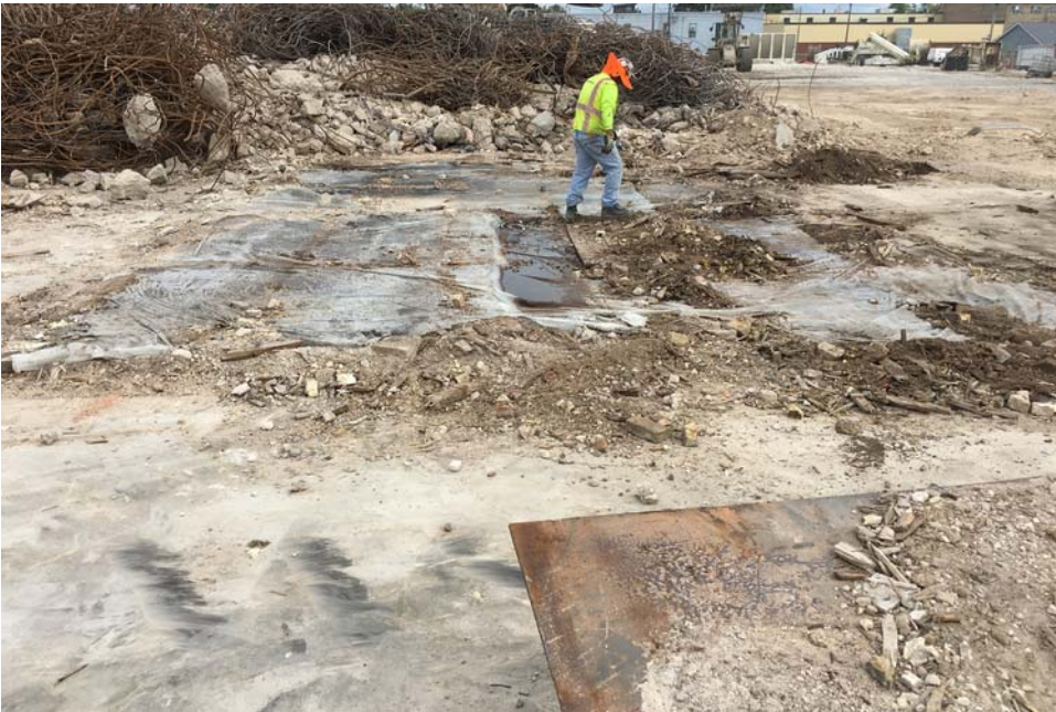
#16 - Plywood cover removed from Area 8
