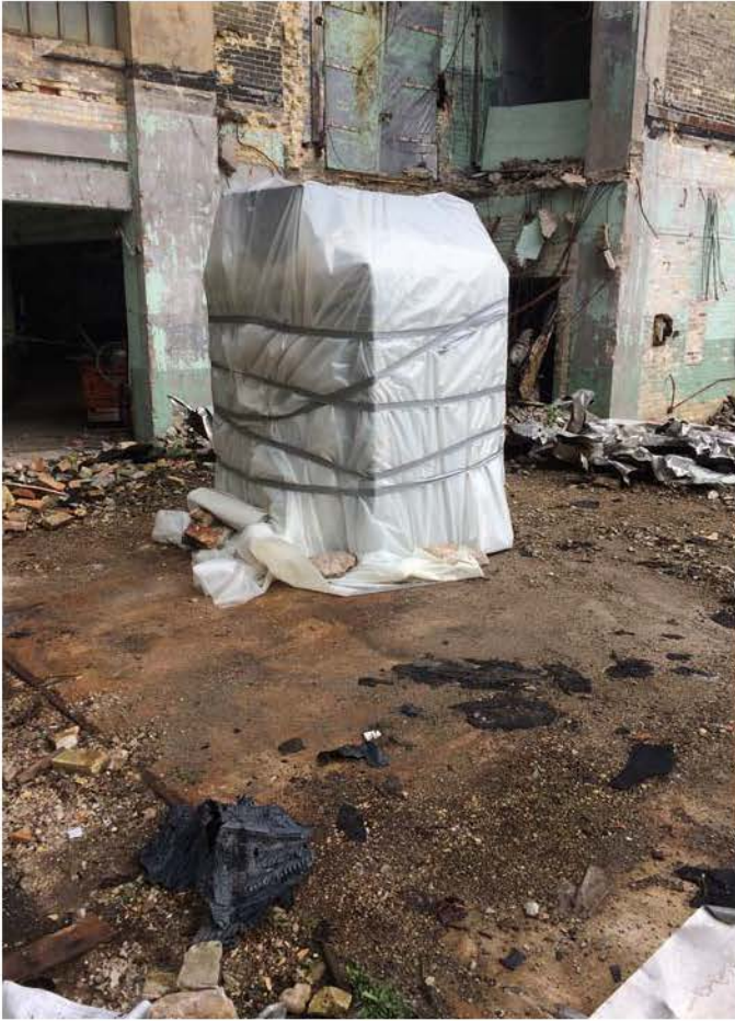
#1 - Removal and packaging of transformer components by Area 8
