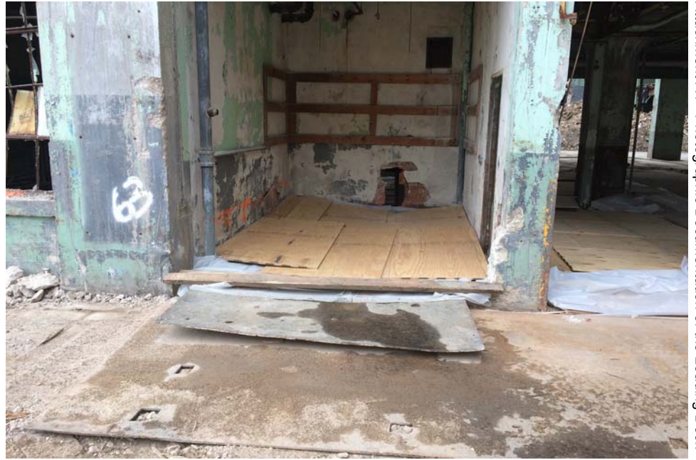
#13 - Temporary cover installed in the Loading Dock
