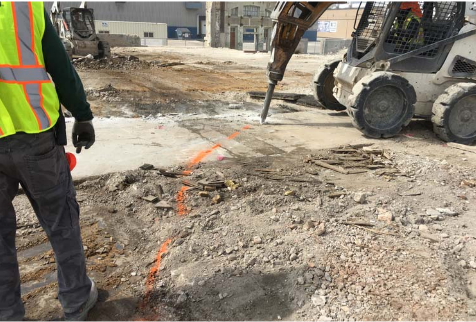
#16 - Marking and breaking concrete for removal
