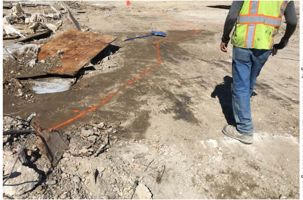
#17 - Marking and breaking concrete for removal
