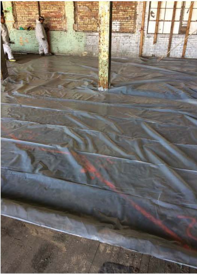
#9 - Installation of temporary cover in Area 8
