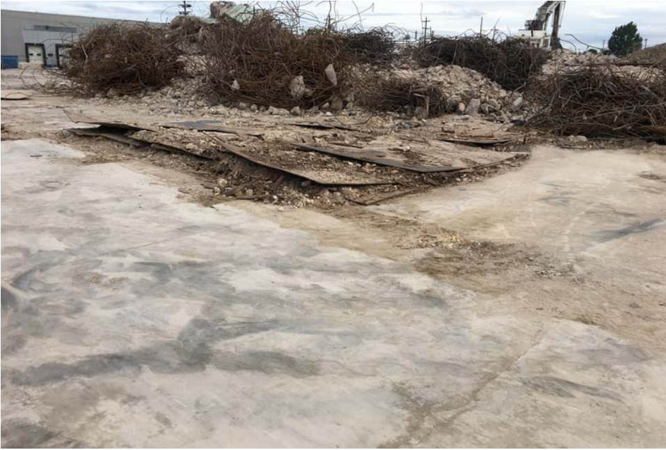
#15 - Area 8 following building demolition, prior to removal
