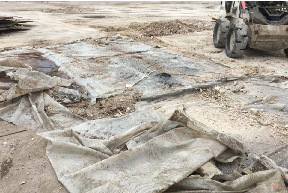
#24 - Breaking concrete from Area 8
