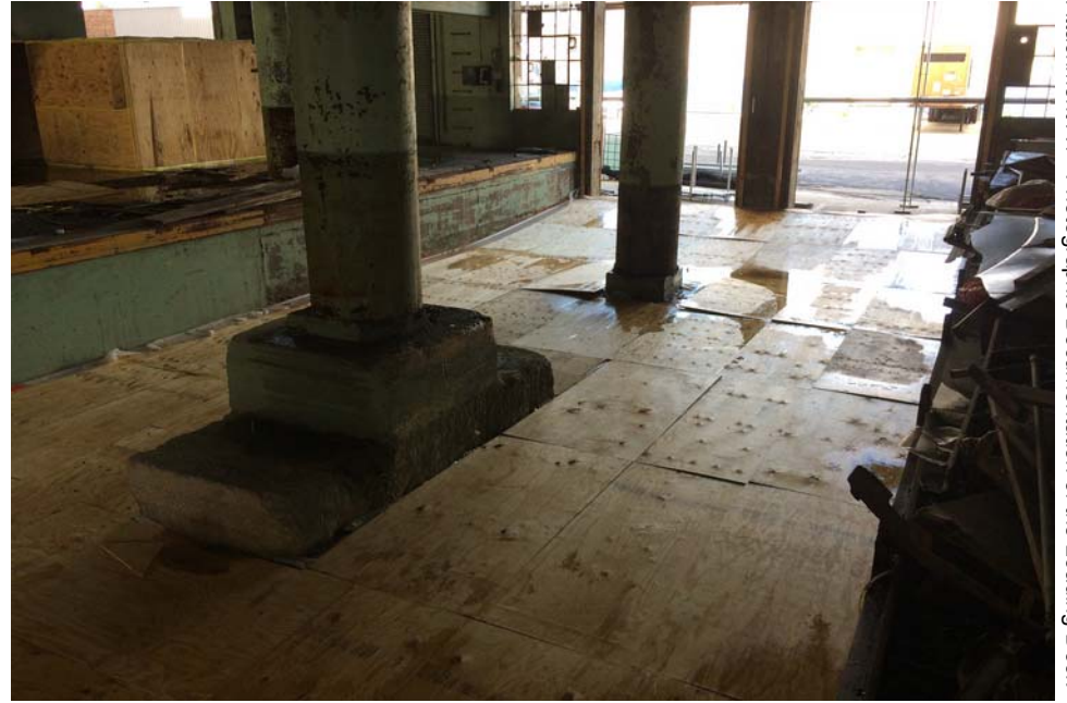
#9 - Temporary cover installed in the Loading Dock
