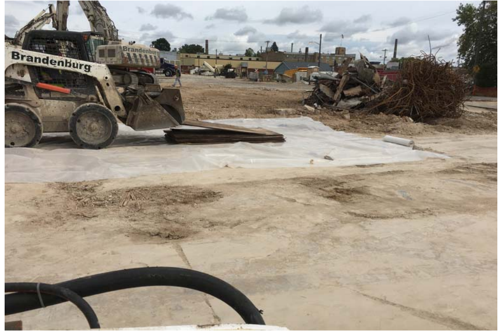
#18 - Wrapping up plywood
