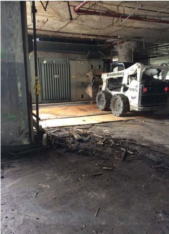
#3 - Removal of transformer from Area 14
