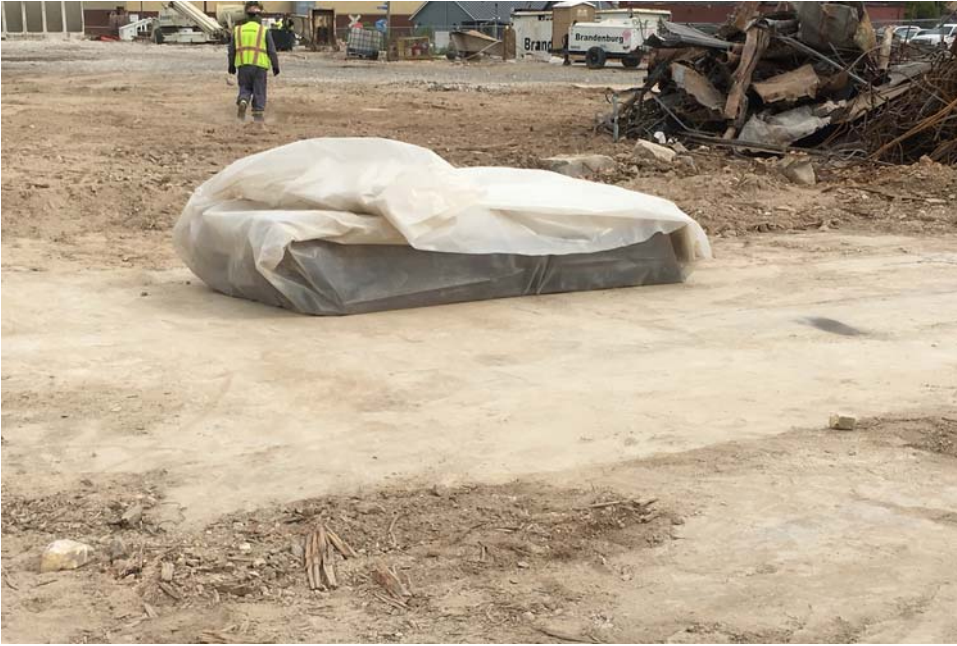
#19 - Plywood cover prepared for offsite disposal
