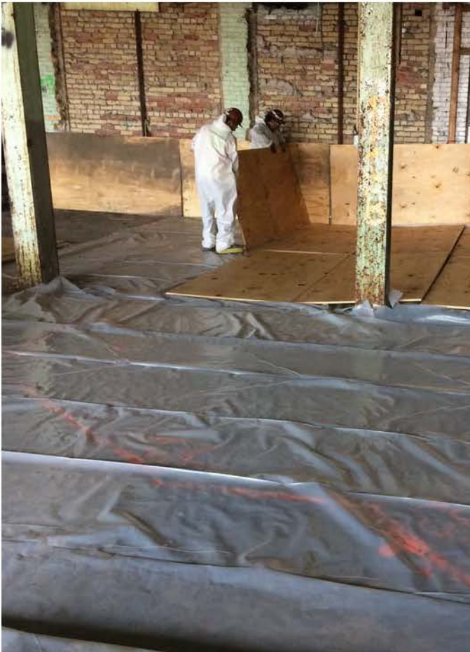
#11 - Installation of temporary cover in Area 8
