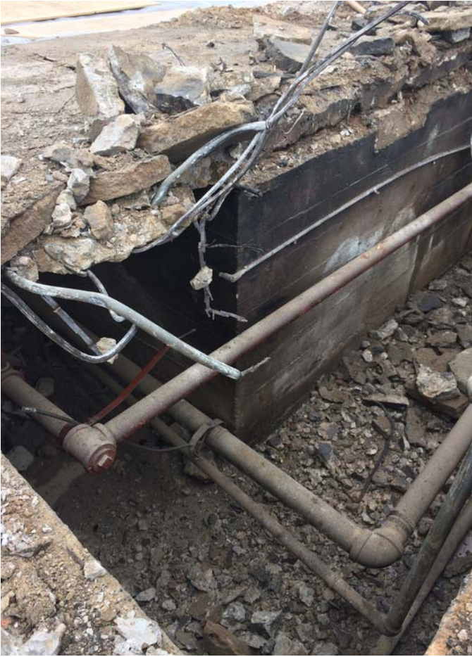
#25 - Utility tunnel adjacent to removal area
