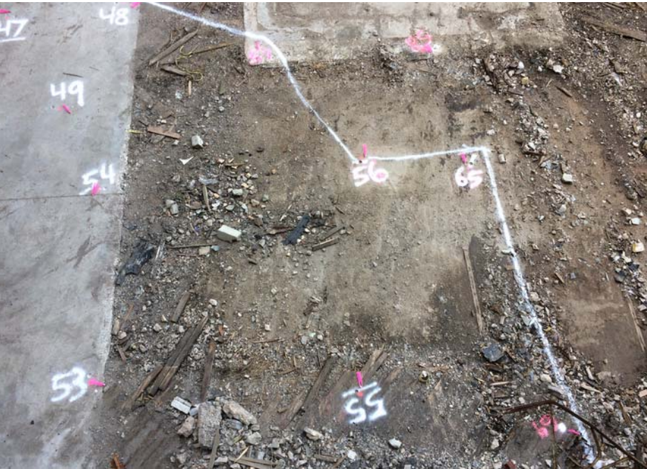
#8 - Delineation of concrete removal area in the Loading Dock
