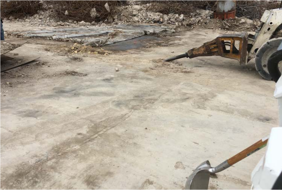
#20 - Breaking concrete from Area 8
