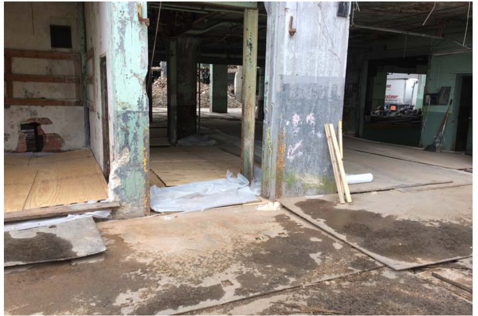
#14 - Temporary cover installed in the Loading Dock
