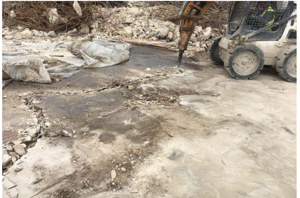
#22 - Breaking concrete from Area 8
