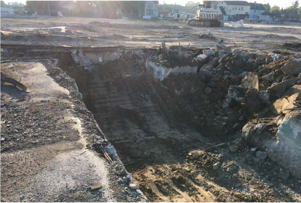
#19 - Demolition of loading dock ramps
