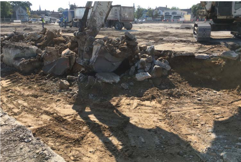
#20 - Removal of concrete debris
