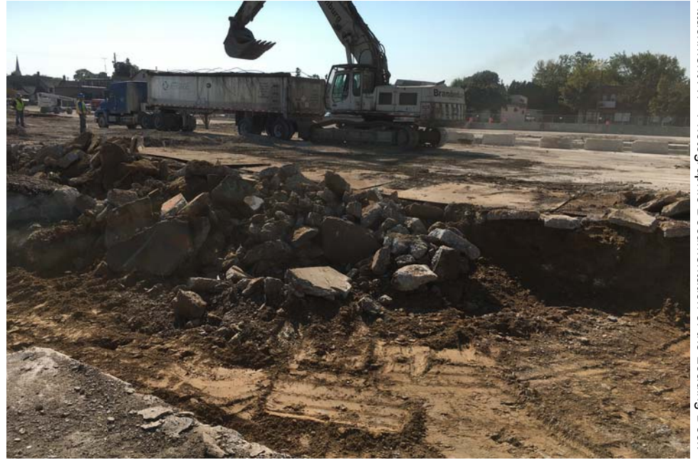
#21 - Loading Heritage truck for transport to landfill
