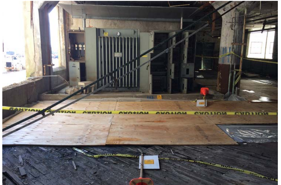
#2 - Temporary cover in Area 14, prior to transformer removal
