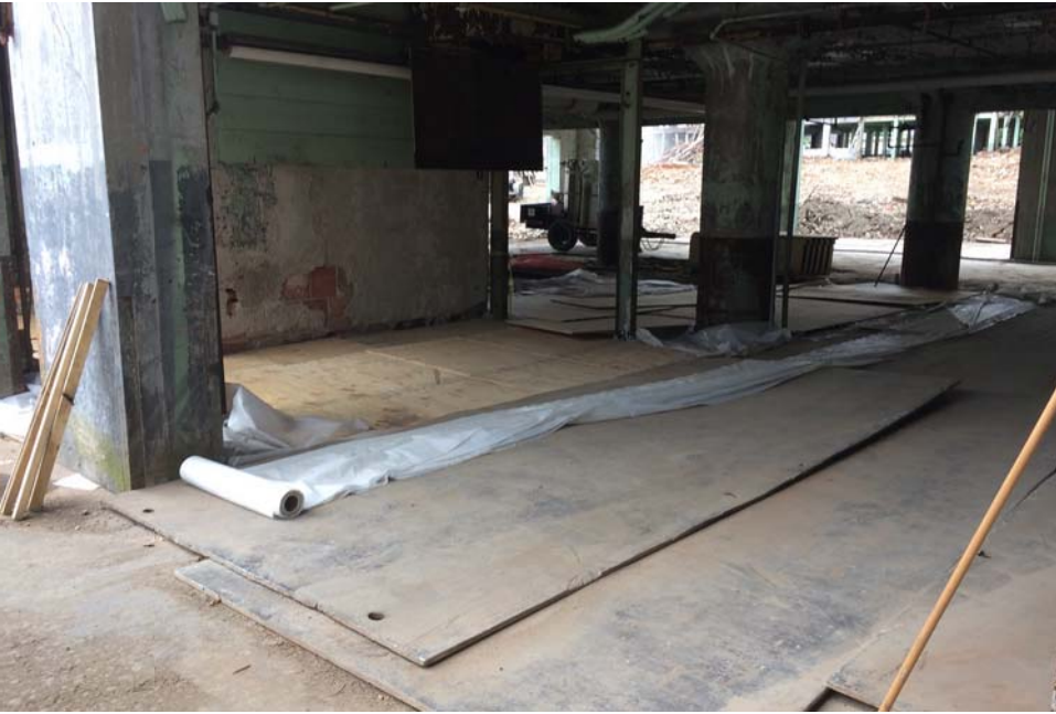
#15 - Temporary cover installed in the Loading Dock
