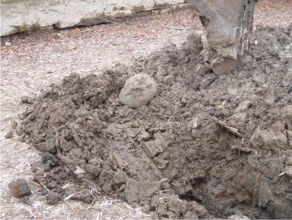
Photo #15. Test Pit #2, note large cobbles beneath the sediment.
