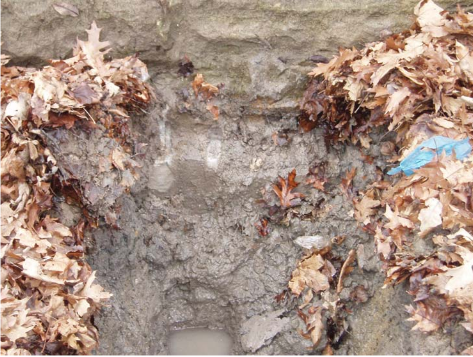
Photo #17. Test Pit #5, retaining wall excavation.
