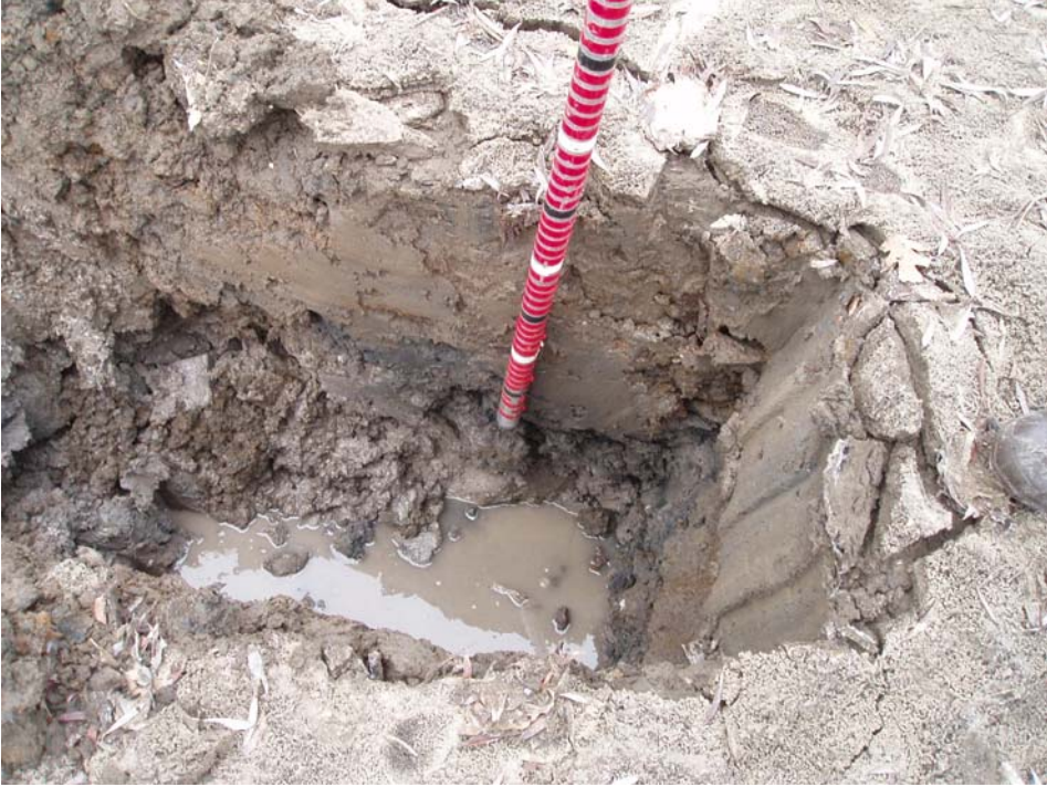
Photo #9. Test Pit #1, south end of Embayment out from retaining wall. White lines are feet.
