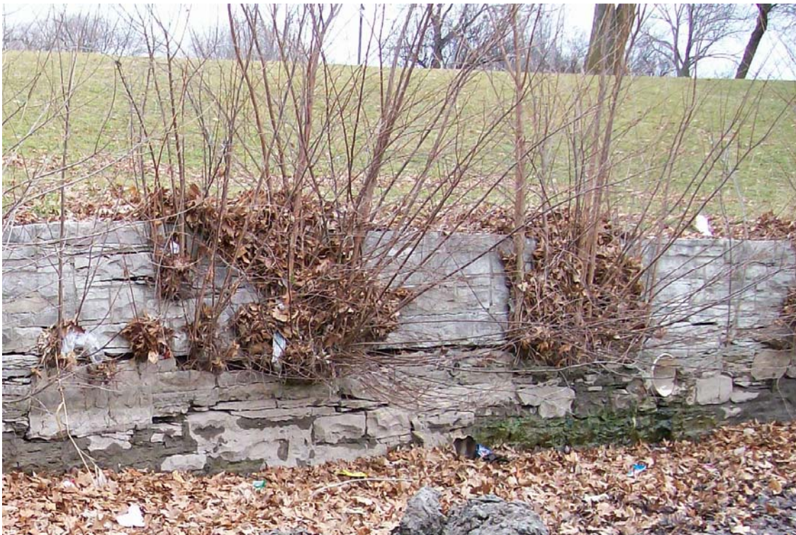
Photograph 2: at north end of wall
