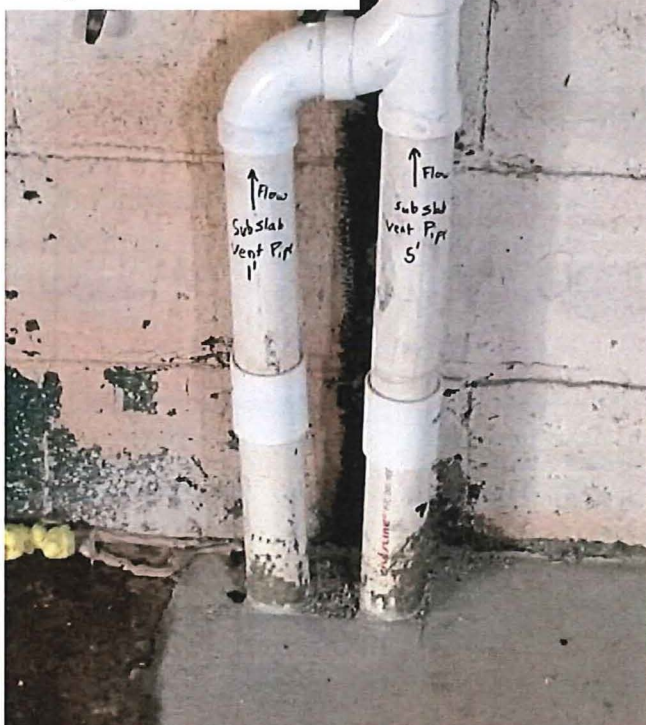
Detail of Subfloor Piping located on Building North Wall, showing connection to Piping that extends through Roof to Fan
