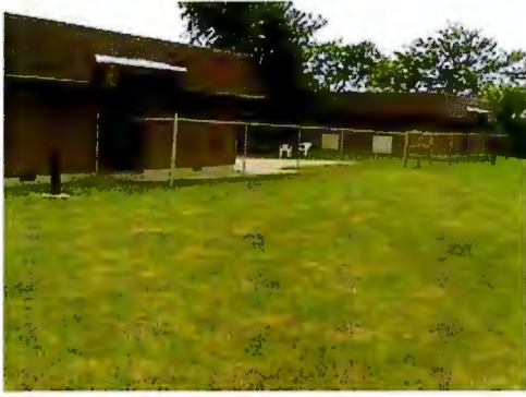
Photo 1 – Health Care Center – Pre-Demo
