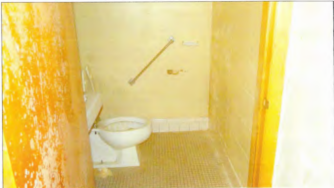
Photo 22: Restroom in Unit 2.
