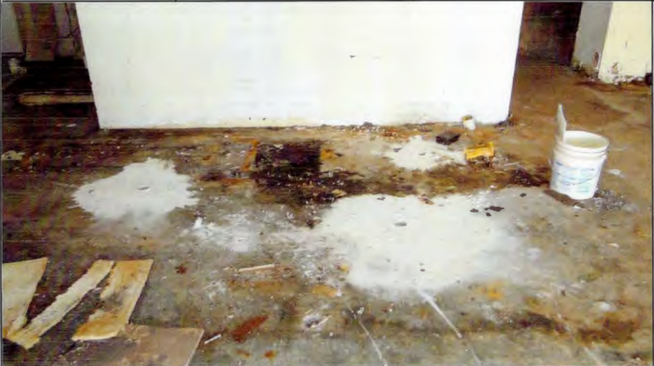
Photo 13: Floor in Unit 1, where dry cleaning machines were located.
