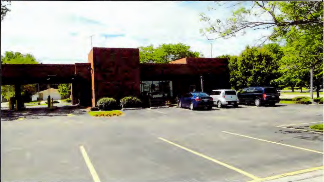
Photo 5: Building to the south of the North Main Street property.
