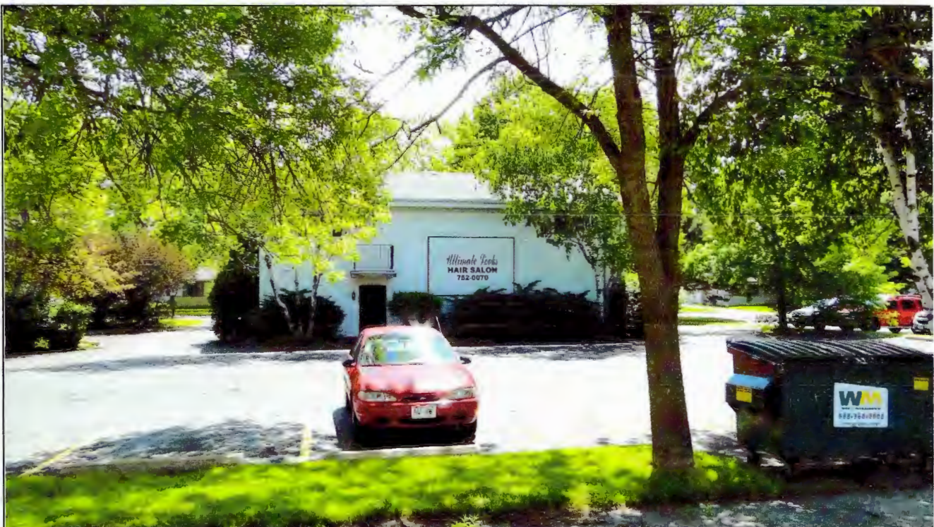
Photo 6: Building east of the southern half of the North Main Street property.
