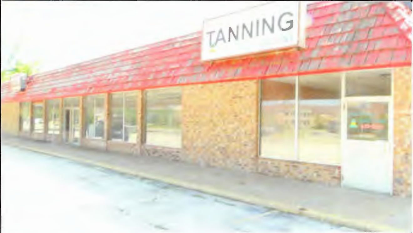
Photo 1: View of front (west side) of building.
