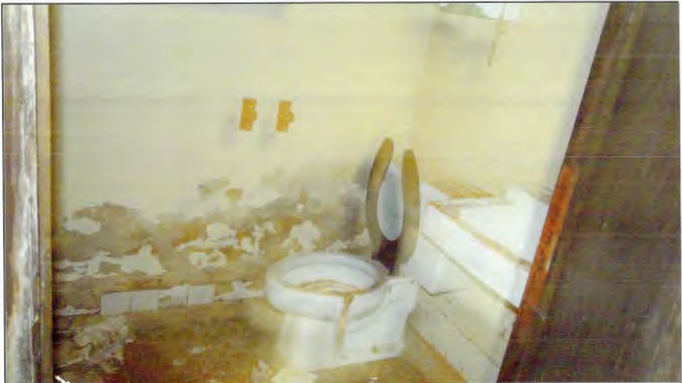
Photo 14: Restroom in Unit 1.
