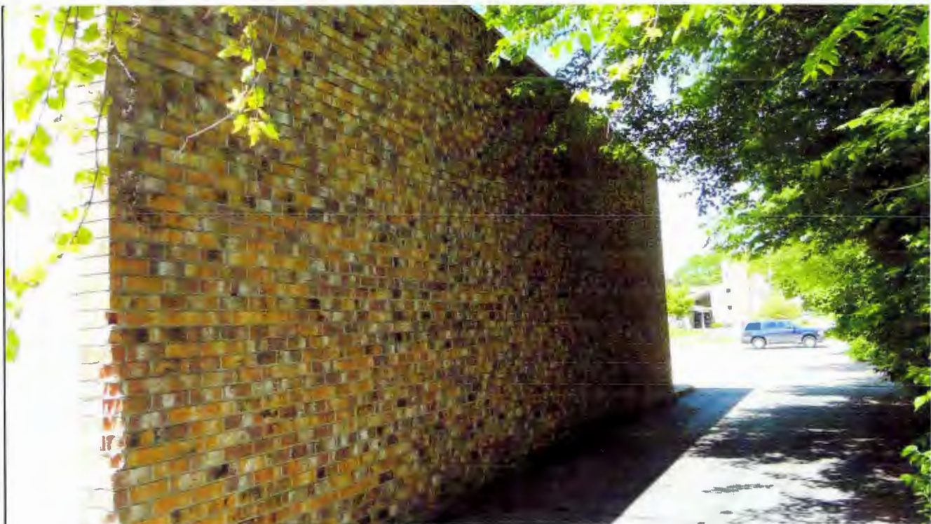
Photo 4: North side of building.
