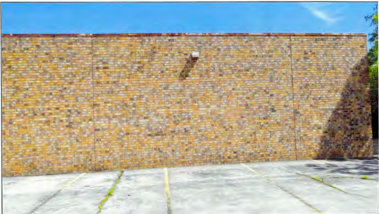
Photo 2: South side of building.
