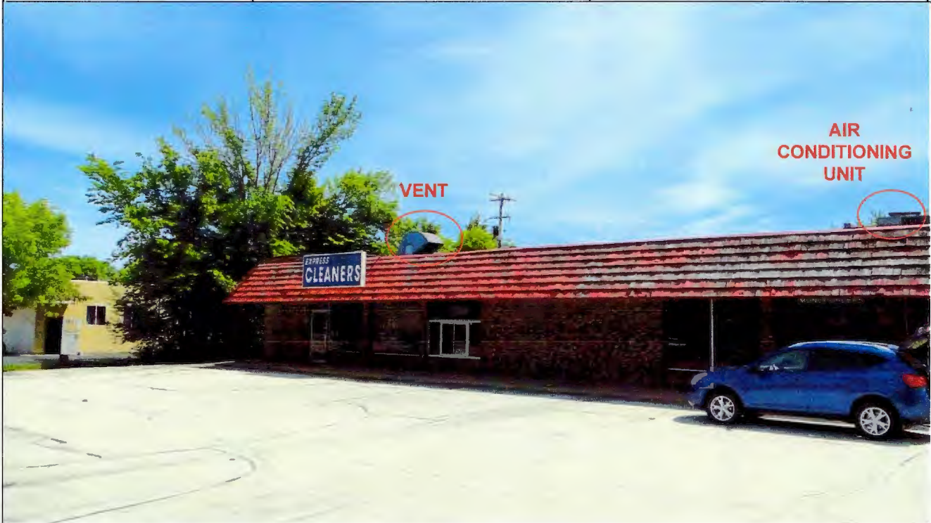
Photo 11: Roof vent and one of three air conditioning units.
