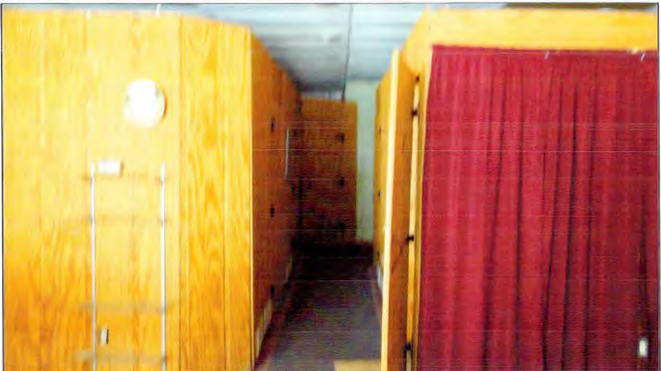
Photo 26: Hallway in Unit 3.
