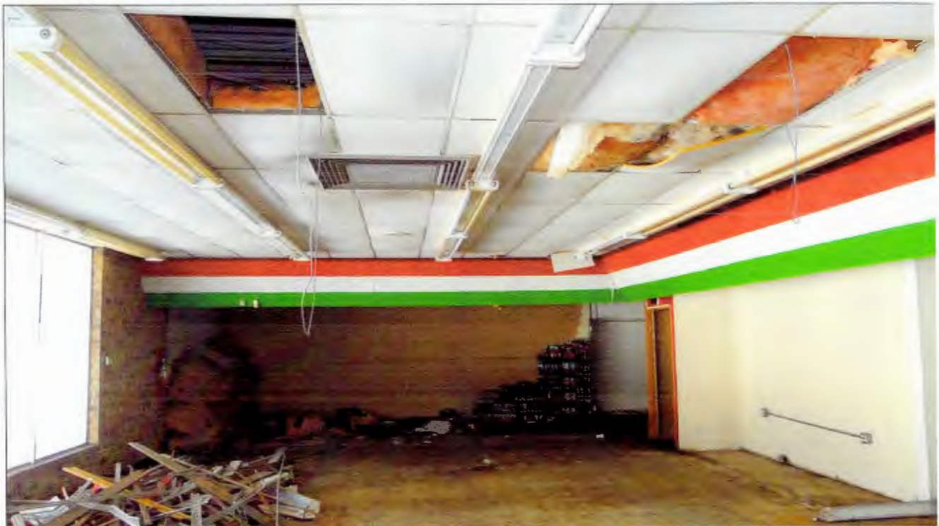
Photo 18: Interior of Unit 2 (former convenience store), looking north.
