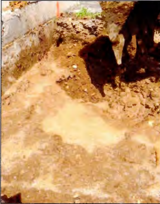
Photo 17. The chemical reaction occurring upon treatment with Cool-Ox™ included bubbling and foaming as the solution was blended with soils. [Photo taken looking northwest]
