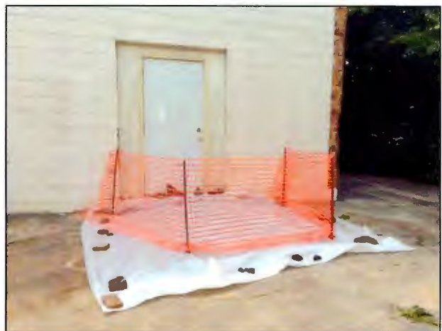
Photo 20. The area was secured by plastic sheeting over treated soils and fencing around the perimeter. [Photo taken looking northwest]
