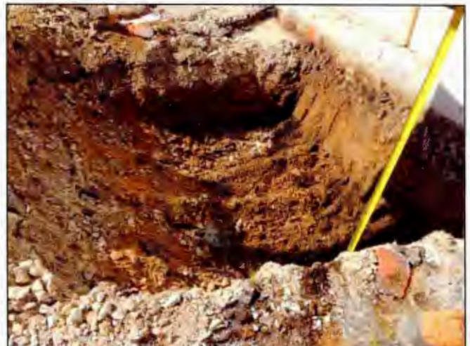
Photo 12. Upon removal of the upper section of soil, a soil sample was collected from the soil pile utilizing a Terracore™ sampler for analysis of CVOCs. Soil was estimated to be from approximately 2.5 feet below surface. [Photo taken looking south]
