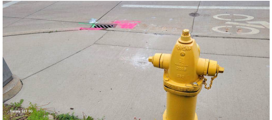
Location of boring B-16 in the sidewalk on Cecil Street on the northwest corner of Cecil and South Commercial Street.
