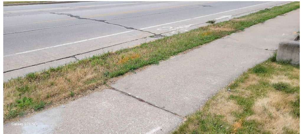
Location of boring B-23 is visible on the lower left-hand side of the photograph. The boring was placed in the sidewalk due to the presence of utilities in the terrace.
