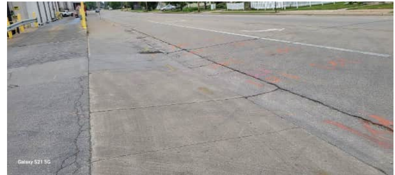
Proposed location of boring B-12 (not completed due to utilities)
