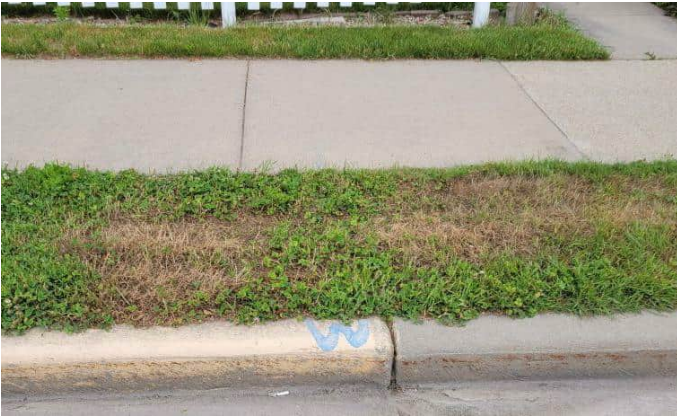
Location of boring B-7 in the terrace to the left of the water lateral.
