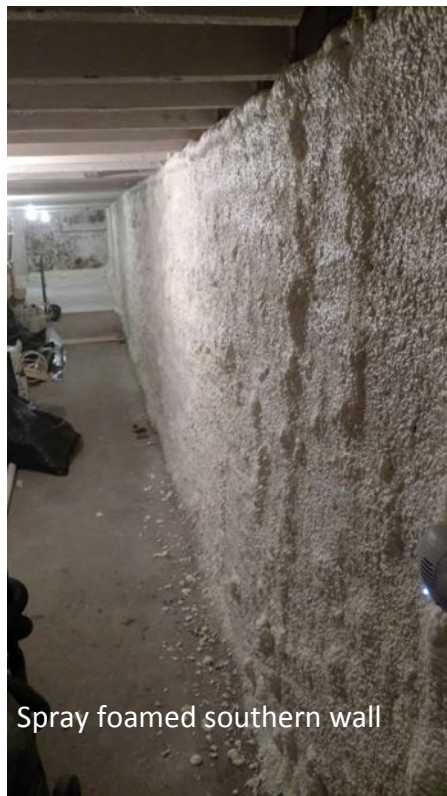
All box headers on southern wall are sealed with 2 in foam board and spray foam
