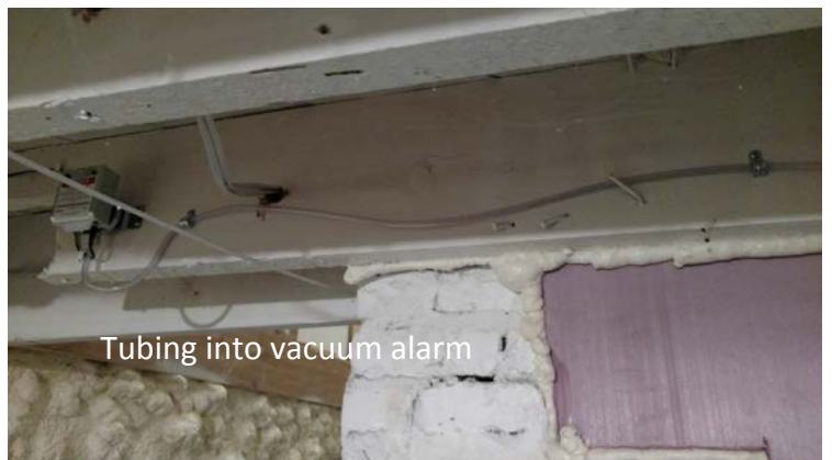
Crawl space sealed with 2in foam board and spray foam
