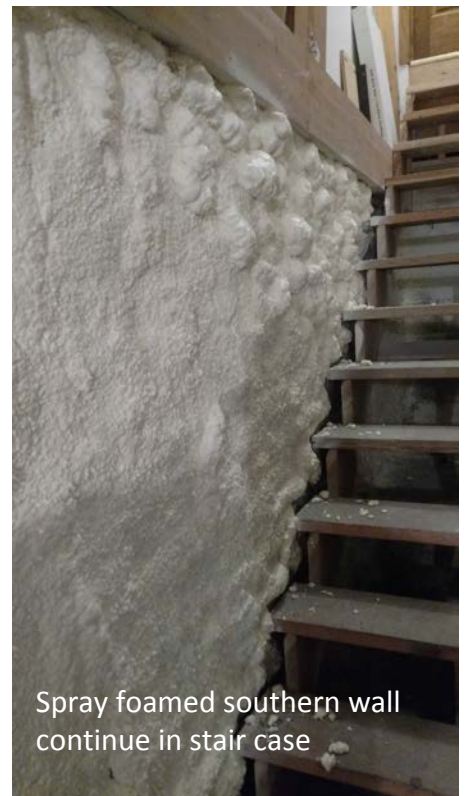
All box headers on southern wall are sealed with 2 in foam board and spray foam
