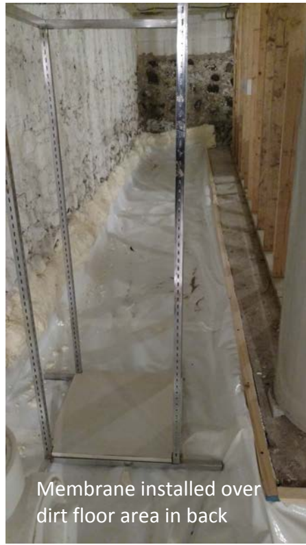
Membrane in back part basement, sealed to the wall with spray foam and anchor to concrete areas with 1 x 2 furring strips
