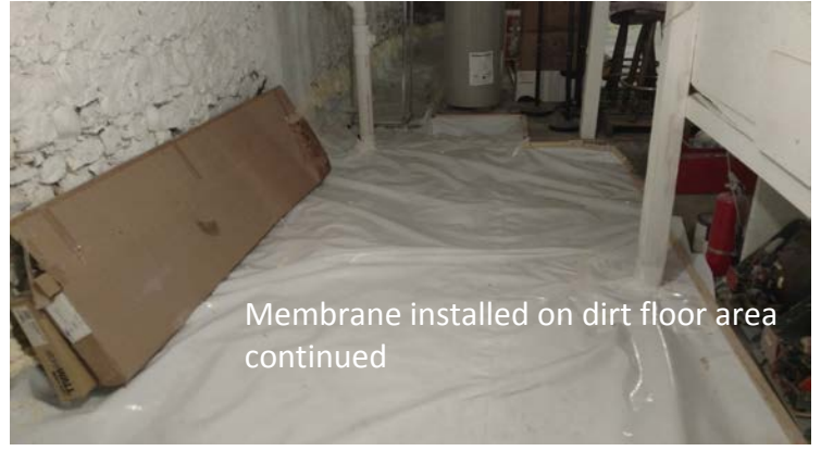
Membrane in back part basement, sealed to the wall with spray foam and anchor to concrete areas with 1 x 2 furring strips
