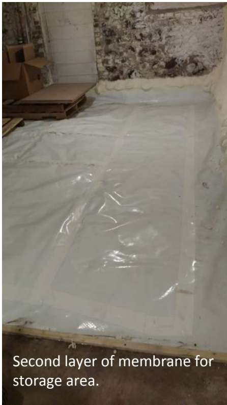
Membrane in back part basement, sealed to the wall with spray foam and anchor to concrete areas with 1 x 2 furring strips
