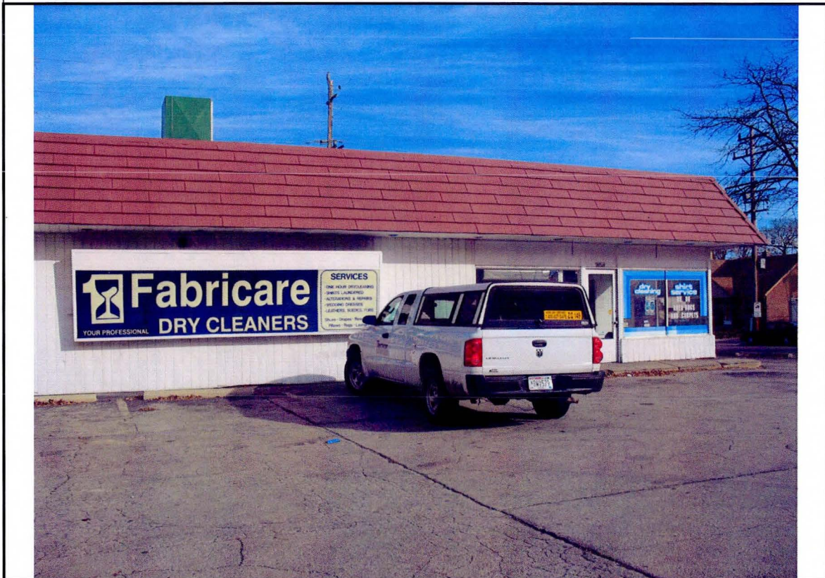
4. View of the south side of One Hour Fabricare from the southwest corner of the site.
