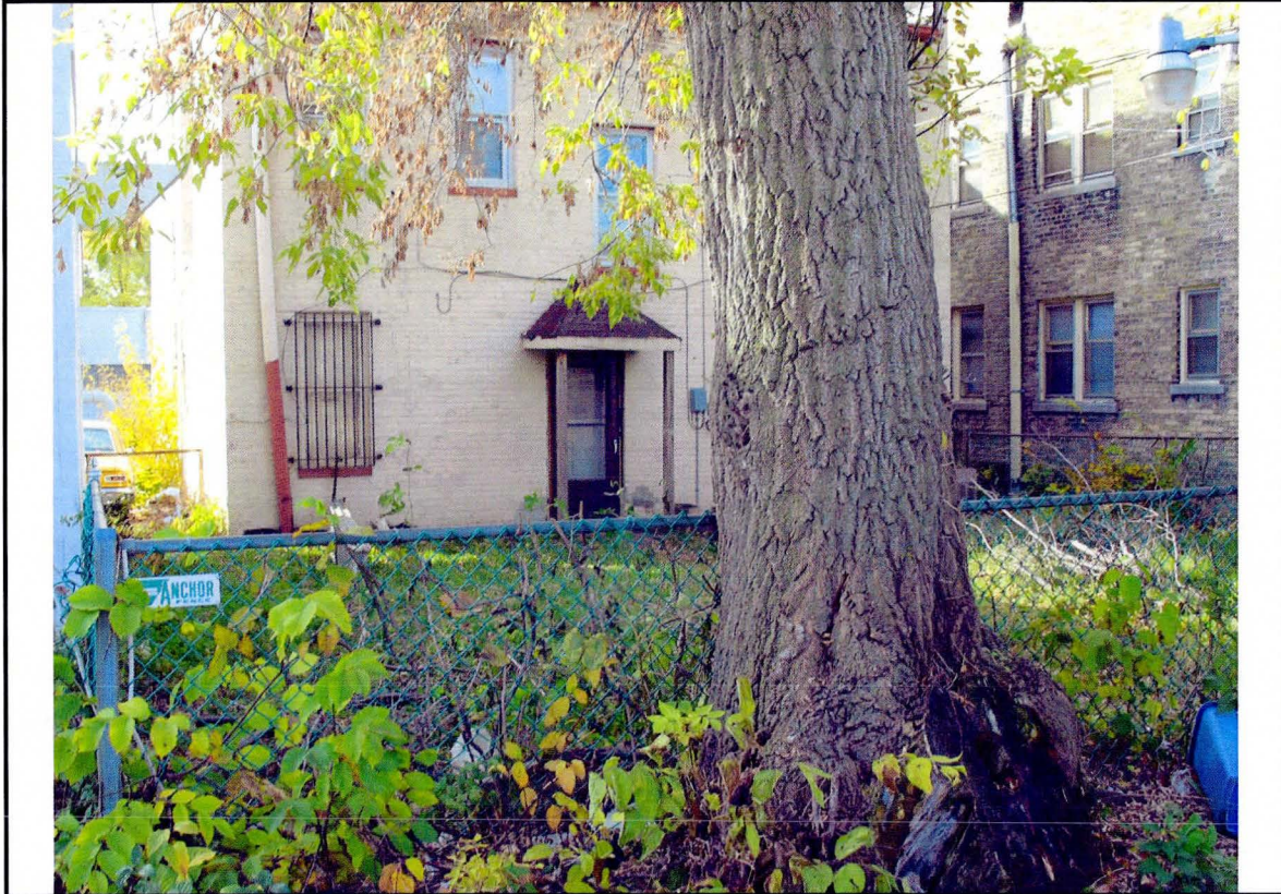
7. View of the west side of the dry cleaner building and the adjacent property to the west of the site.
