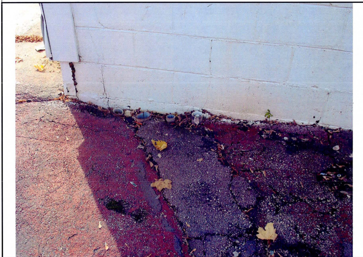
16. View of pipes adjacent to the north side of the dry cleaning building.
