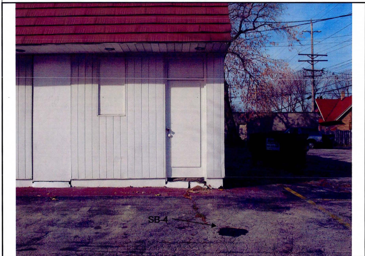
14. View of soil boring SB-4 to the east of the dry cleaning building.
