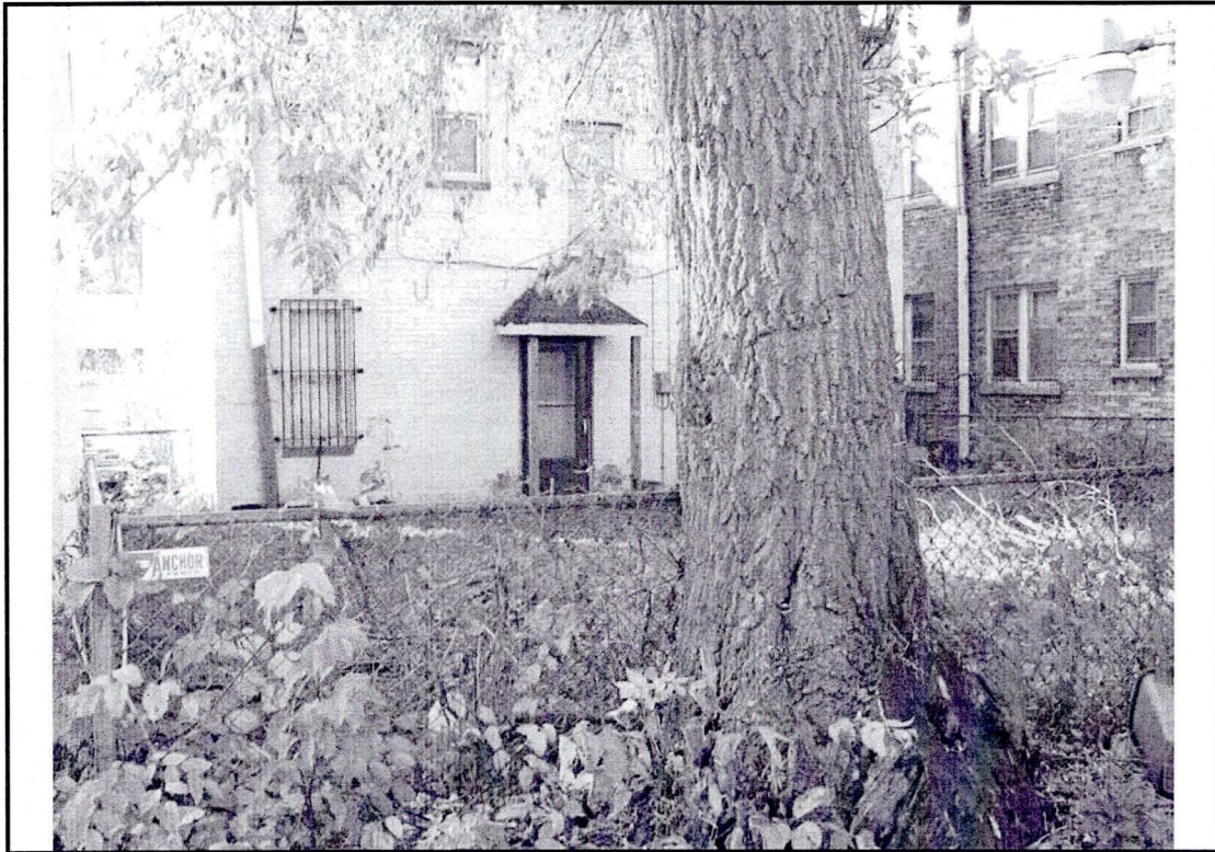
7. View of the west side of the dry cleaner building and the adjacent property to the west of the site.
