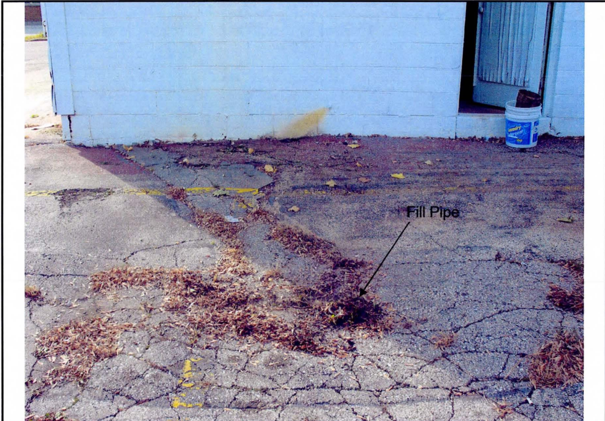
15. View of the fill pipe to the underground storage tank to the north of the dry cleaning building.
