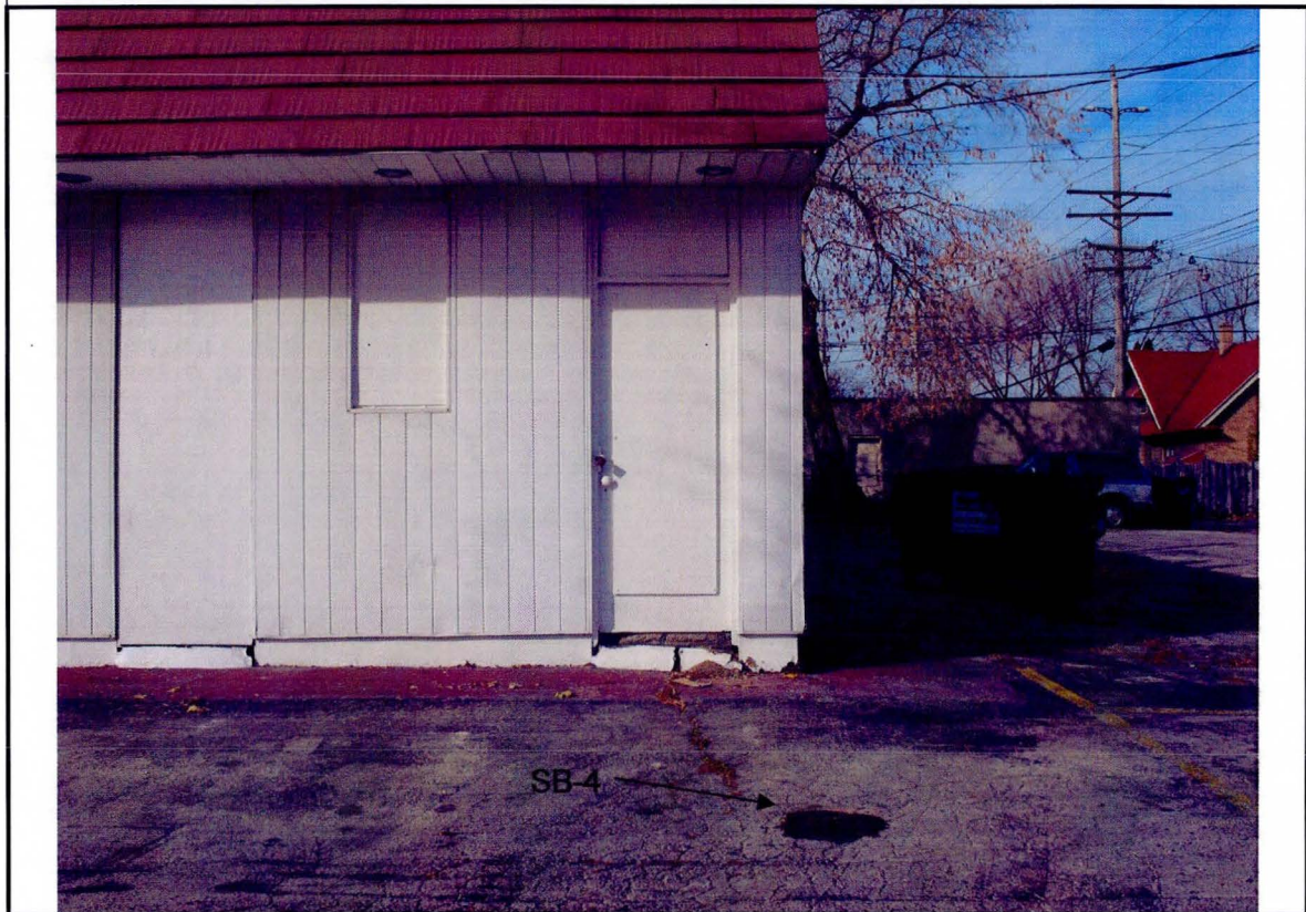
14. View of soil boring SB-4 to the east of the dry cleaning building.
