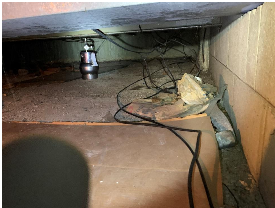
Photo #6 Indoor Air Vapor Sampling in crawlspace at 3119 N. 47 th Street residence.
