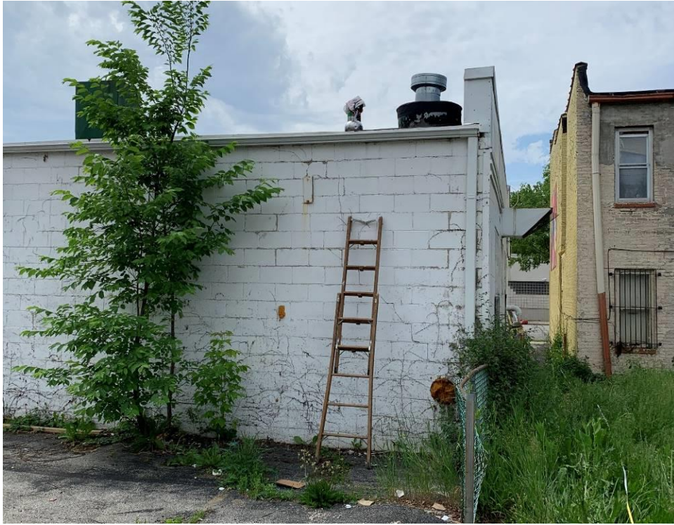
Photo #7 Ambient Air Sampling on roof of 4704 W. Burleigh Avenue building.
