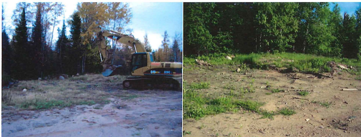
One truckload (17.03 tons) of material was removed from an area located on the northwest side of the property at which historical burning is known to have occurred. Before and after photos.
