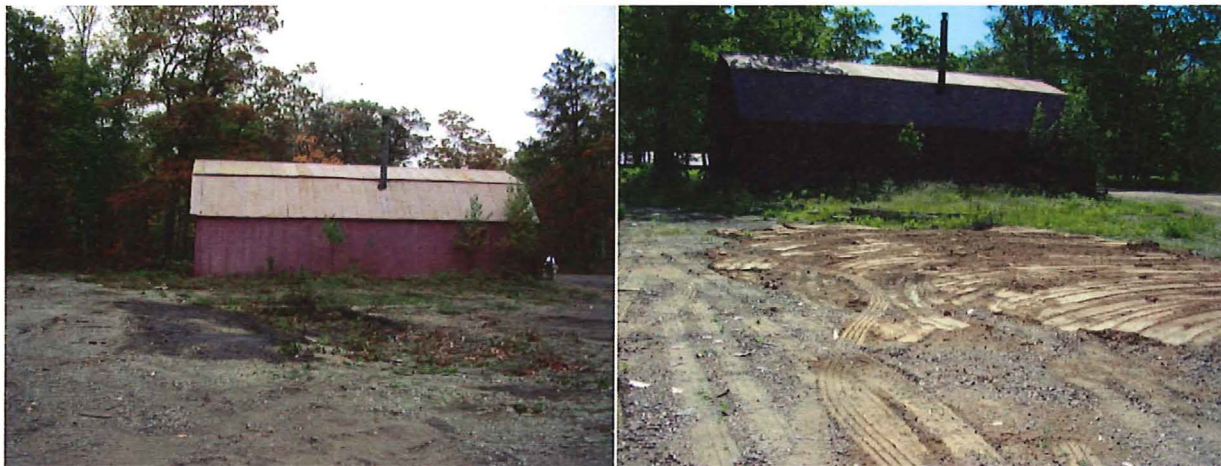
Surface staining located north of Area H and east of Area E was excavated in October 2007. Clean fill was brought to this area in June 2008. Photo on the left is before, on the right is after.
